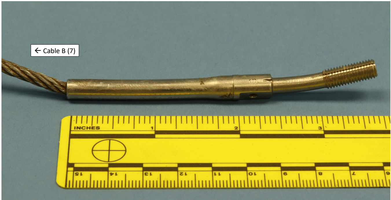
Figure 2: A photograph of the threaded end terminal of cable B (7) as received, which exhibited bending deformation.
