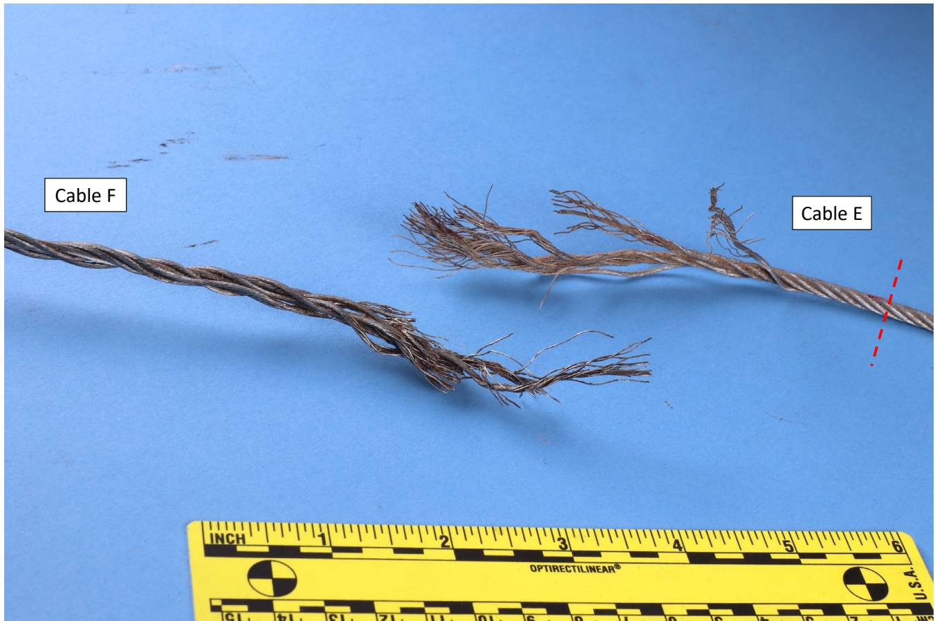
Figure 11: A photograph of both sides of fractured cable 26. Strands and wires were raveled and splayed open approximately 4 to 6 inches from the fracture surface. The red dashed line indicates the approximate location of a section cut made in cable E to facilitate closer exam of fractured wires using SEM.
