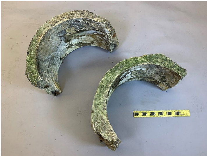
Figure 2. Two halves of 1-foot in length concrete exterior coating that separated on-site from the west end of the pipe segment.
