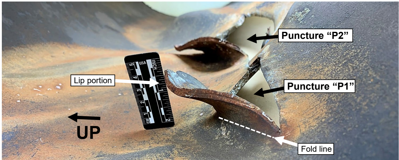
Figure 21. View looking east at the Inner surface of the pipe showing puncture "P1" in the foreground and puncture "P2" in the background, after cleaning. Dashed line indicates a fold line at the base of the lip.
