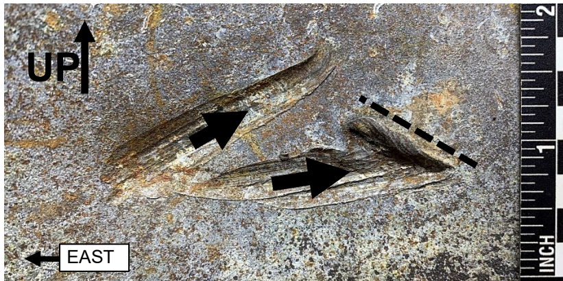
Figure 16. Close-up photograph of the outer surface of the pipe in the area of dent “D1” showing two major gouges located within dent, after cleaning. Arrows indicate general direction of metal flow. Metal flow terminated in the general area indicated by a dashed line.
