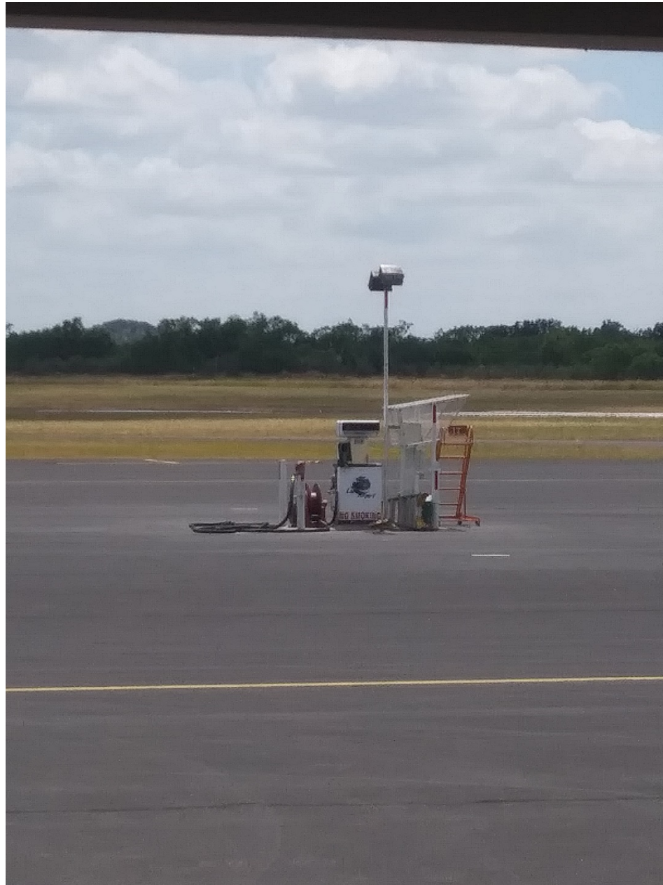
Photo 13 - Supplied photo of the fuel farm ramp at AQO.
