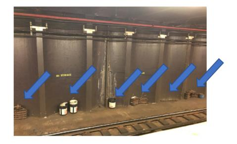
• 6/21/21 Inspection: Inspected Jack Arches in City Hall Station and 8th & Market St. Station. The vast majority of the Jack Arches were clear of objects. No more than one contained an object. All conditions were acceptable.
