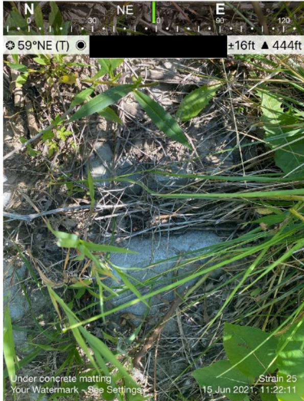
Photo 12. Concrete matting over pipeline.
