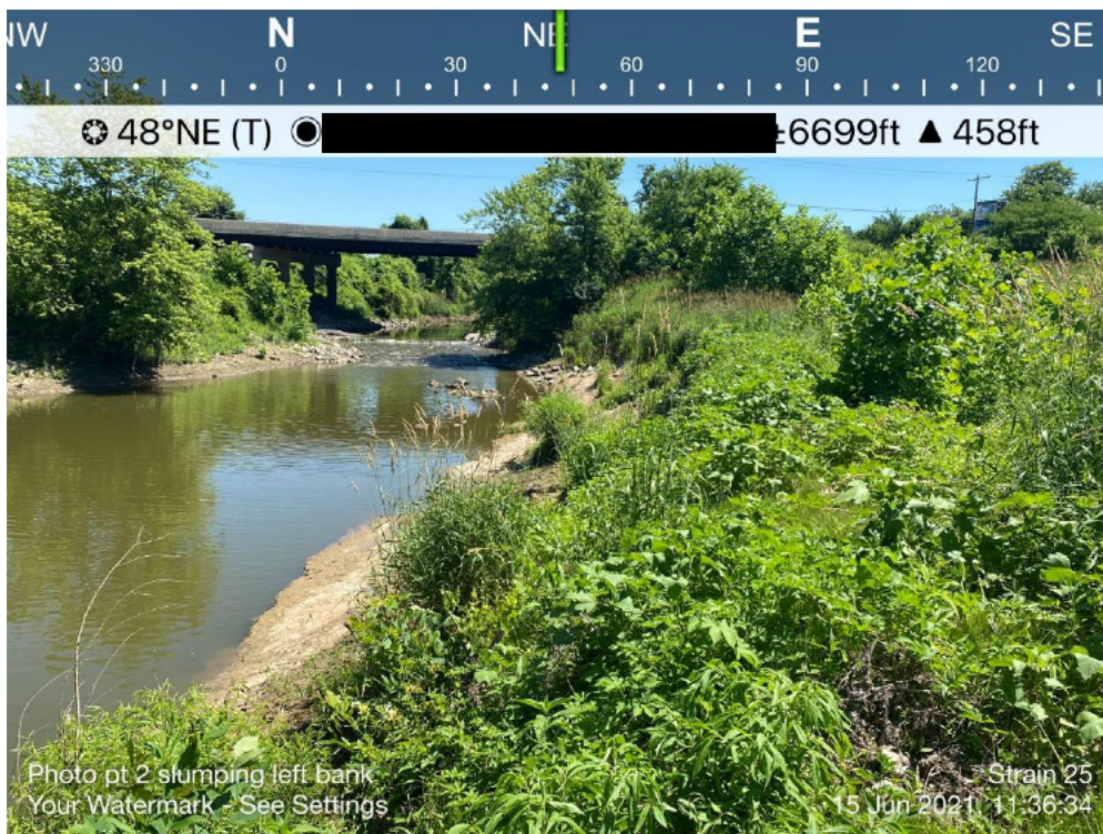
Photo 8. Photo location 2 looking upstream and at slumping on left bank.
