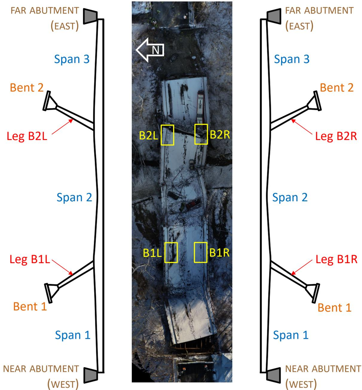
**Figure 2.** Plan view composite photo of the collapsed structure relative to the elevation view schematic, with each leg identified.
