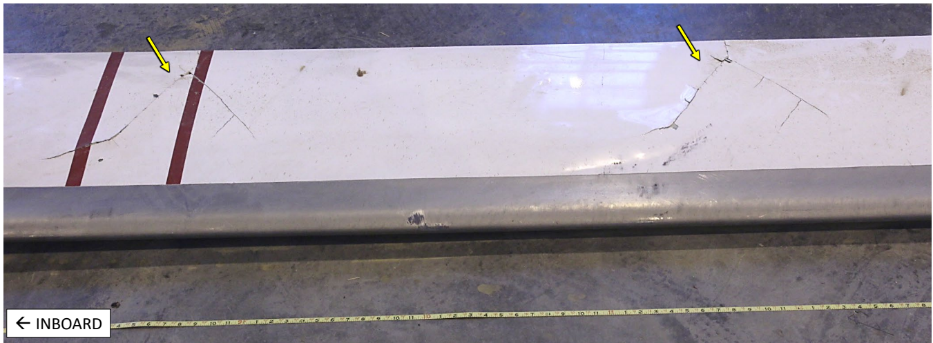
Figure 10: Photograph of inboard branched cracking sites, indicated by yellow arrows, observed on the red blade, lower skin.
