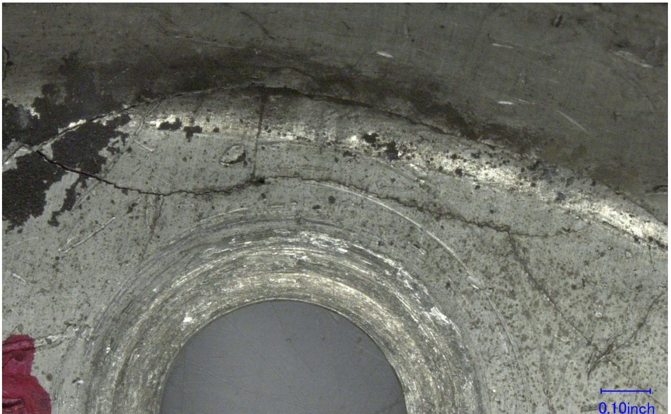
Figure 14 – Closer view of crack #5 from the forward side.
