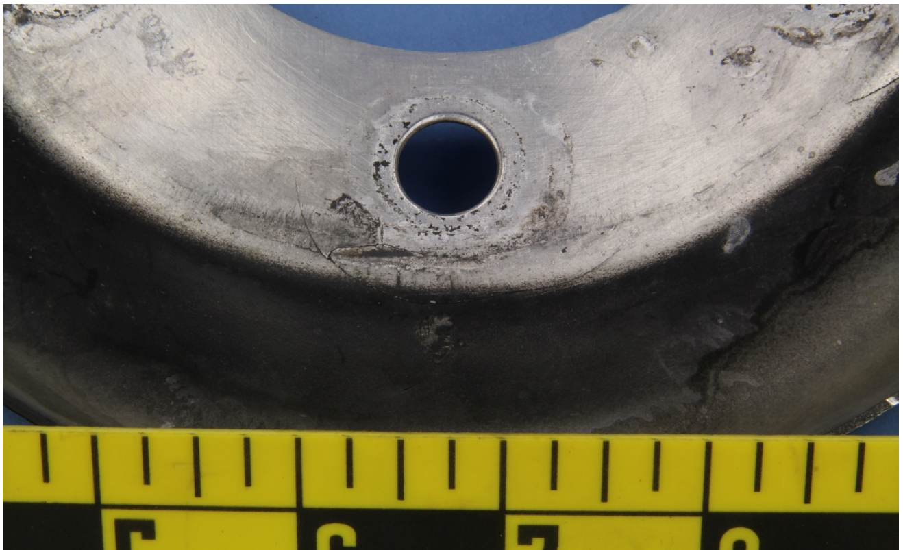
Figure 8 – View of the crack around the bolt hole #5.
