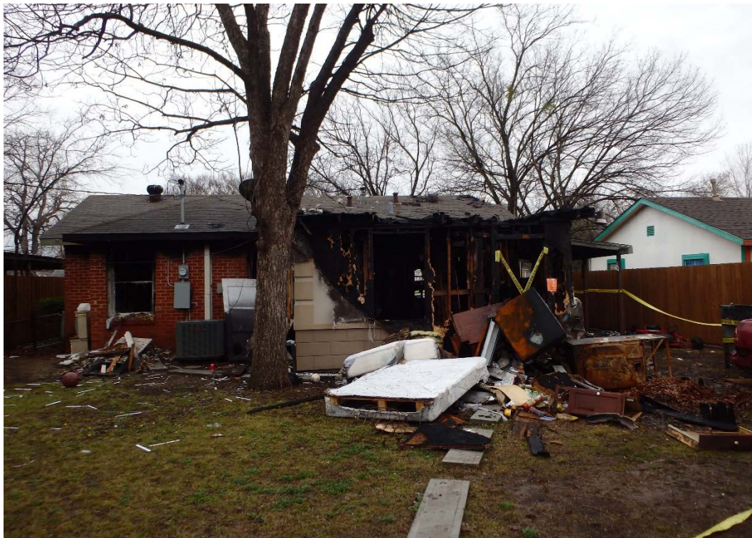
Figure 39. Side C of 3515 Durango Drive. Photograph by DFR, February 2018.
