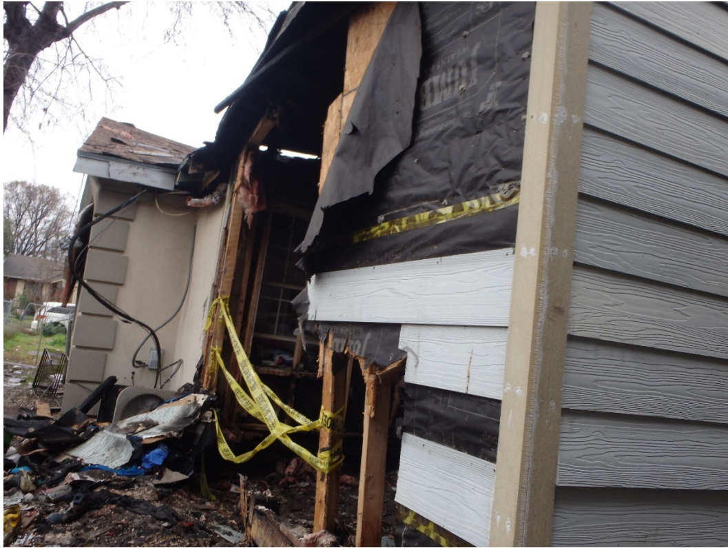
Figure 10. Side D for addition for 3527 Durango Drive. Photograph by DFR, February 2018.
