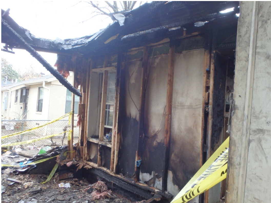
Figure 20. Bedroom wall in addition of 3527 Durango Drive. Photograph by DFR, February 2018.
