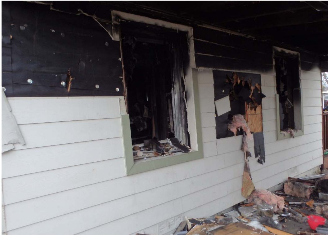
Figure 38. Side B of 3515 Durango Drive. Photograph by DFR, February 2018
