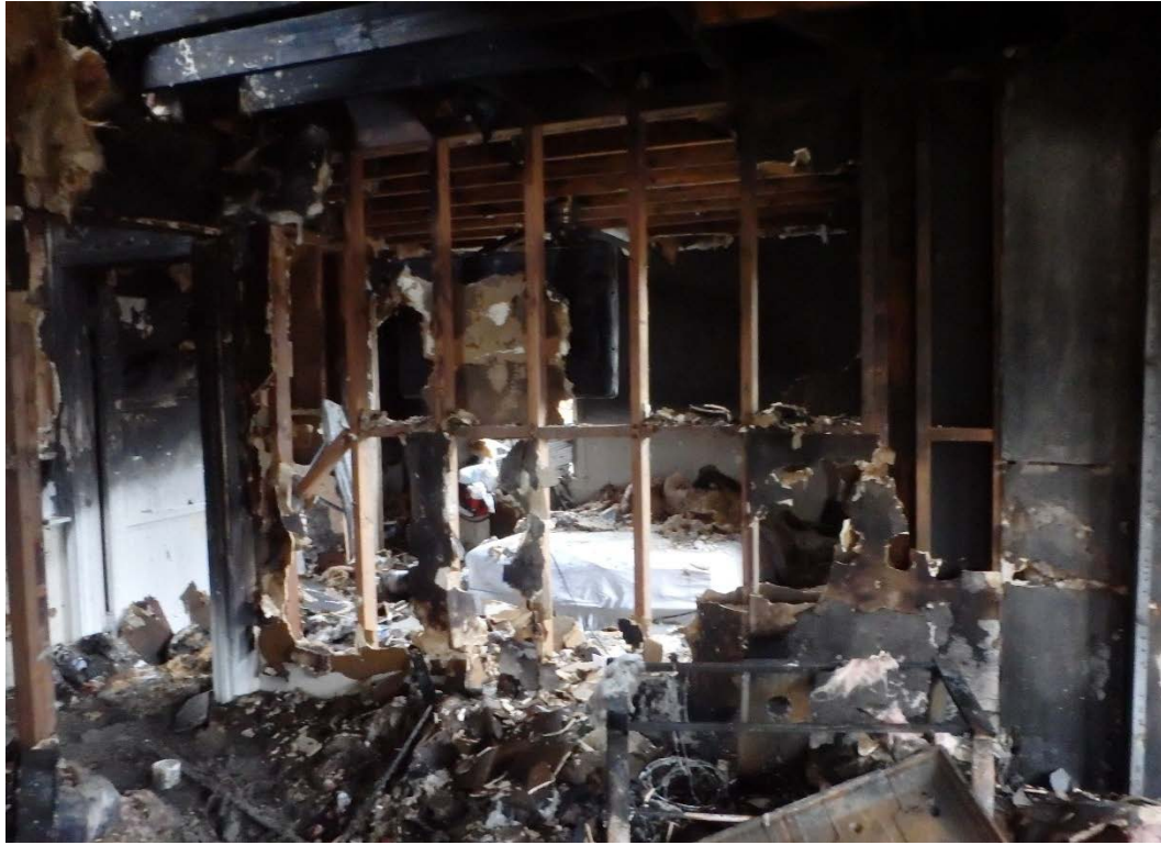
Figure 43. Interior room of 3515 Durango Drive. Photograph by DFR, February 2018.
