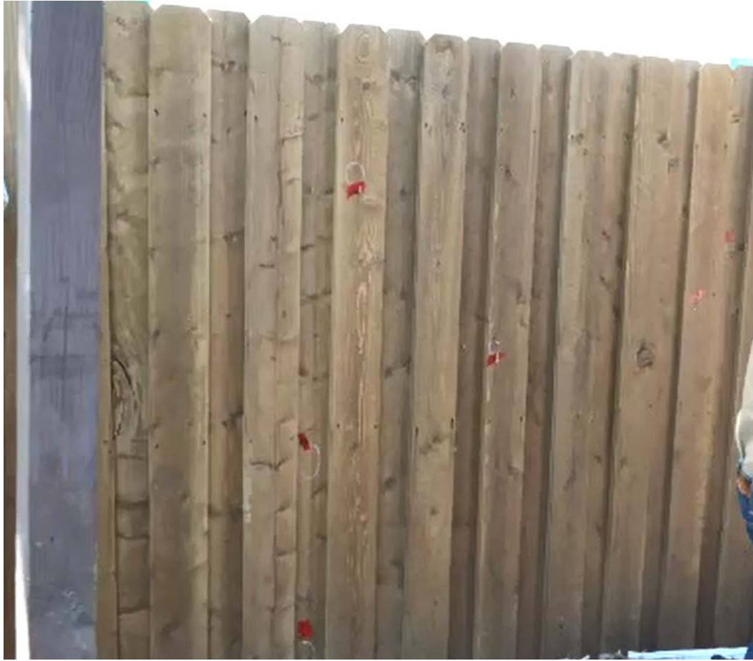
Figure 42. Fence panel with embedded glass located next to the carport for 3515 Durango Drive. Screenshot of video taken by homeowner's representative, April 2018.
