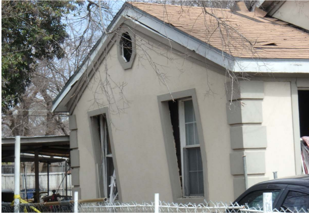
Figure 5. Side B of 3527 Durango Drive. Photo by DFR, February 2018.
