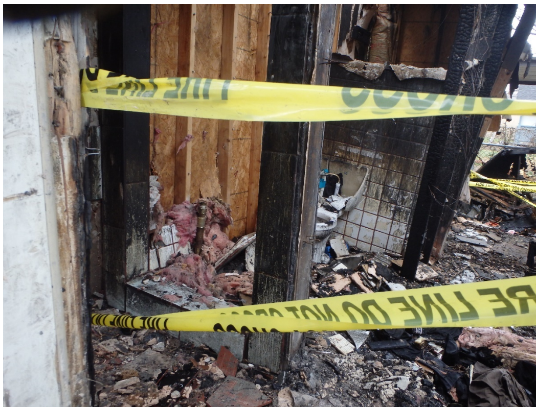
Figure 22. Bathroom in addition of 3527 Durango Drive. Photograph by DFR, February 2018.
