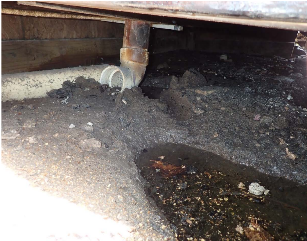
Figure 12. Crawlspace under addition for 3527 Durango Drive. Photograph by DFR, February 2018.
