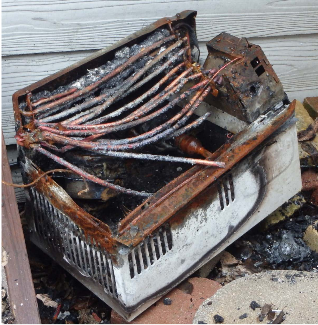
Figure 23. Window air conditioning unit from 3527 Durango Drive addition bedroom window. Photograph by DFR, February 2018.
