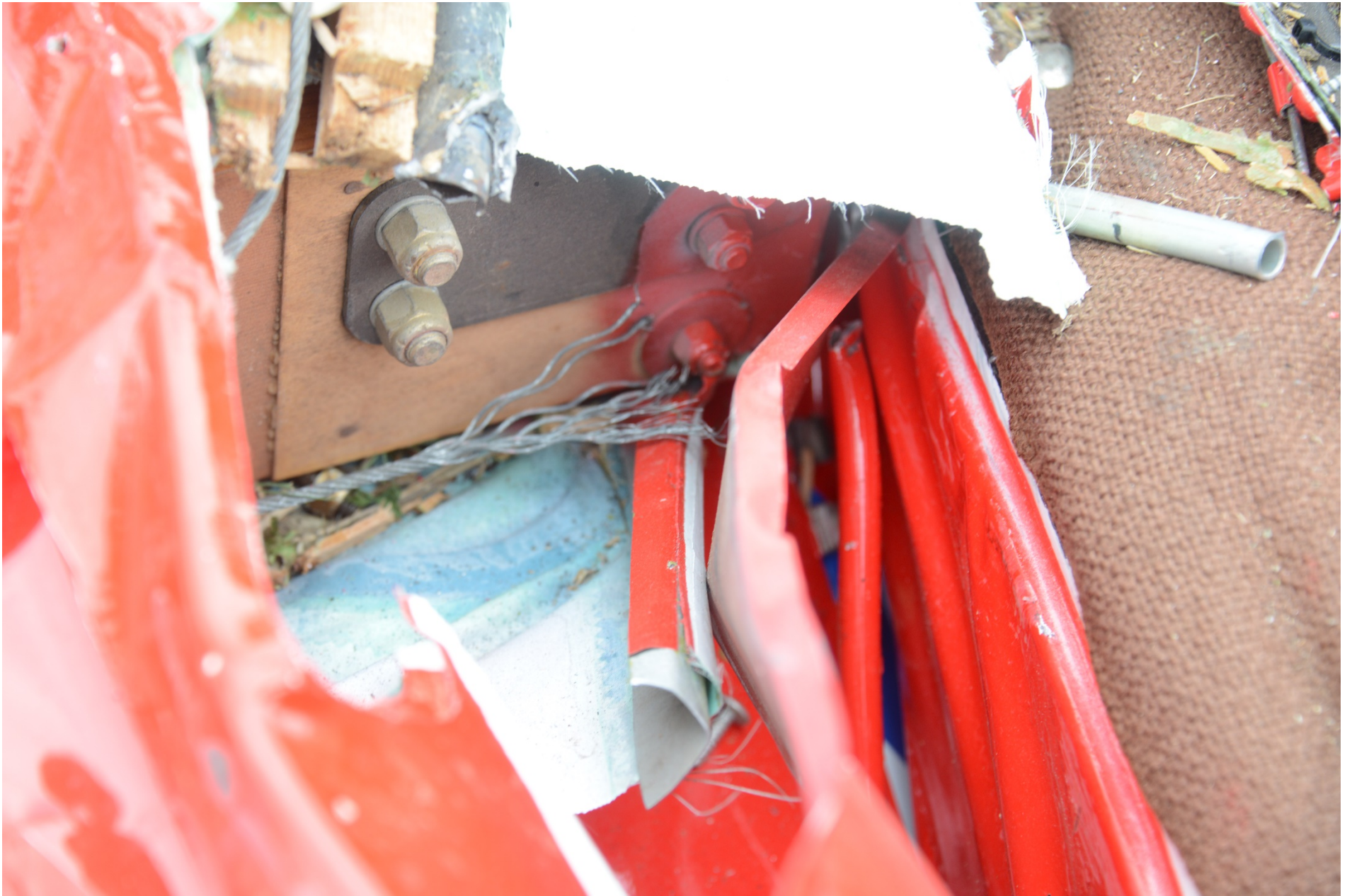
Photo 8 - View of a separated flight control cable exhibiting a broomstraw appearance.
