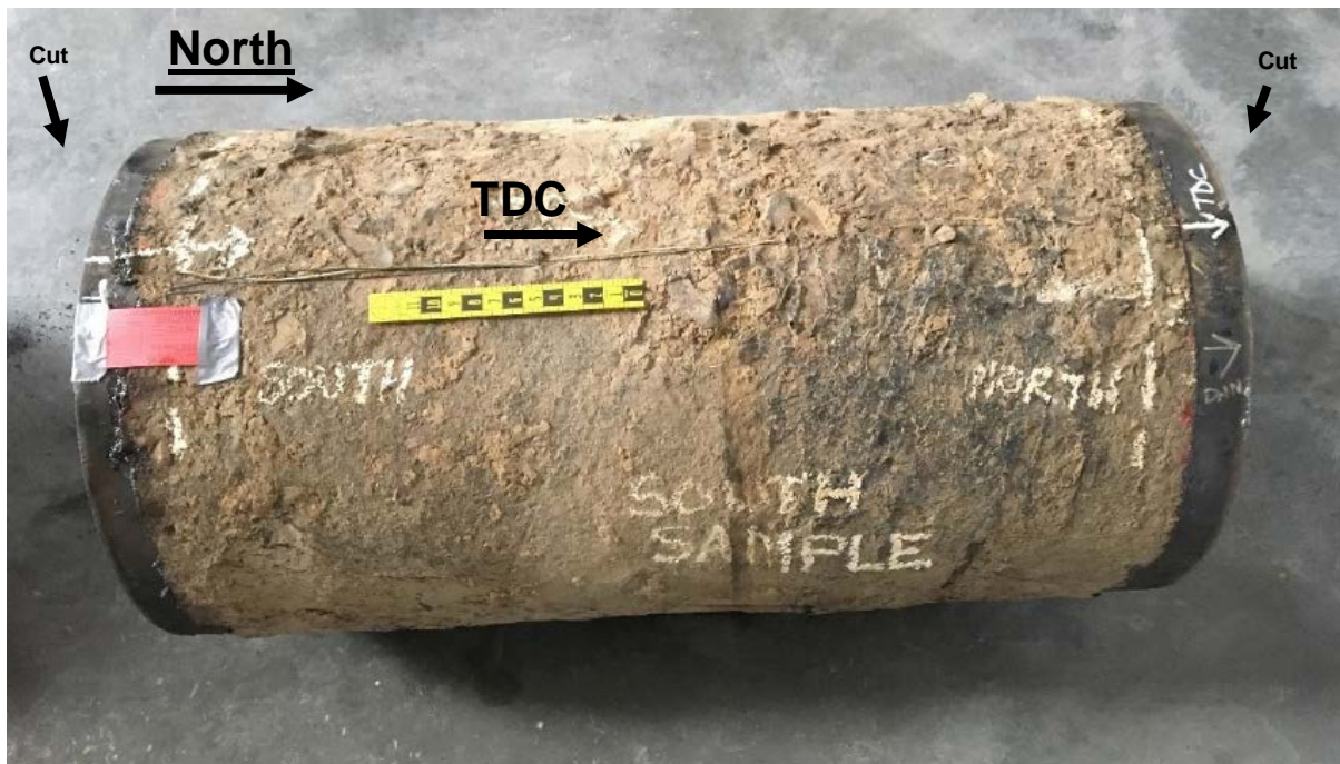
Appendix 3C. As-received 4-foot long ring segments of the pipe that were cut from the pipeline. North sample is shown on the top side of the page and the south sample is shown at the bottom of the page.
