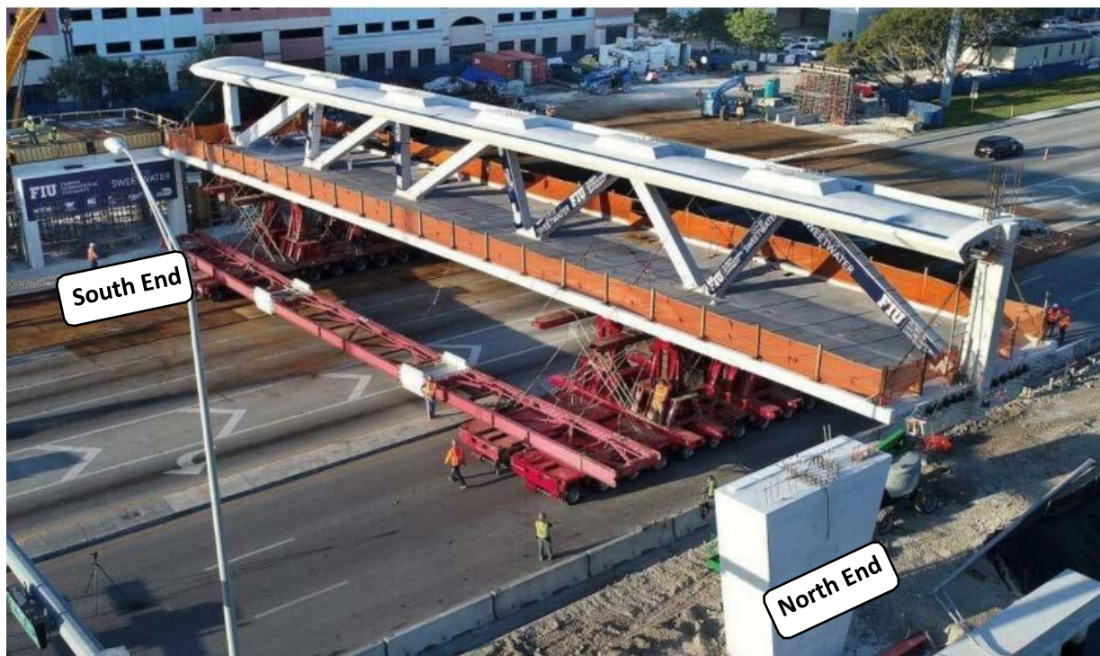
Figure 1. Span 1 of the FIU pedestrian bridge being moved into place
