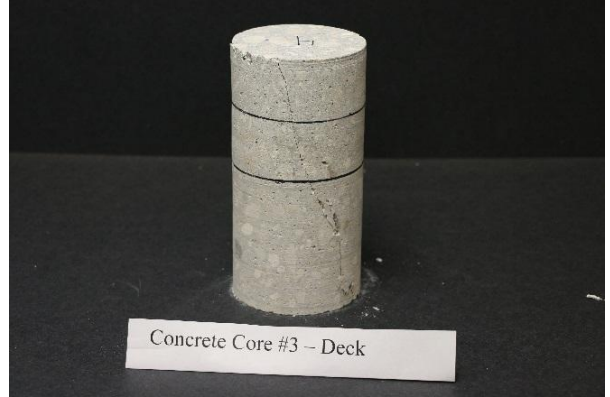
(b) Concrete Core #3 – Deck: Back
