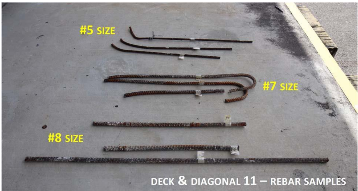
Figure 15: (Top) Photo showing some of the reinforcing bars collected from Diagonal 11 while at the FDOT yard prior to sectioning. (Bottom) Photo showing some of the reinforcing bars collected from the pieces stored at the FDOT yard and sent to TFHRC for testing.
