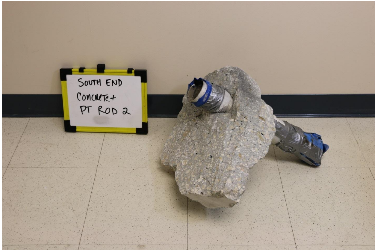
Figure 8. Concrete segment with embedded PT duct recovered from south end of bridge
