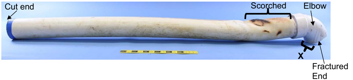
Figure 2. As-received sewer pipe. The fracture in the elbow portion emanated from the outer face in the area indicated by bracket "X". Figure 4 shows another view of the same fracture origin area indicated by bracket "X".
