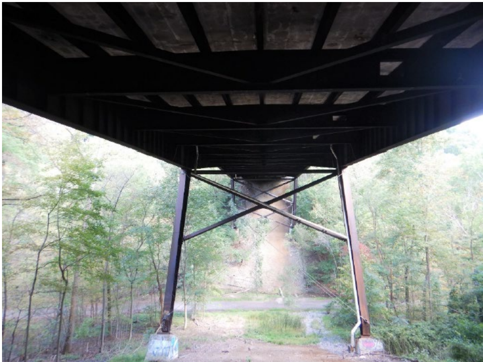
Figure A-6. Bent 1, from the September 2021 report
