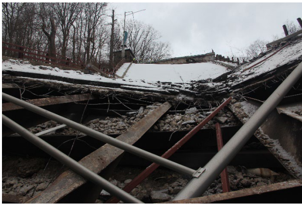
Figure 18. View of demolition removal looking far to near on February 8, 2022.
