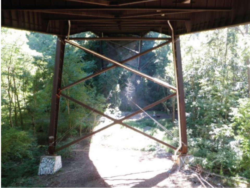
Figure A-5. Bent 1, from the September 2013 report.
