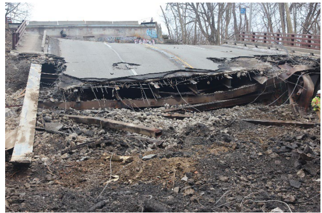
Figure 19. View of demolition removal looking near to far on February 12, 2022.
