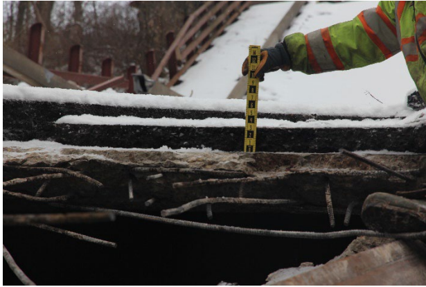
Figure 20. Reference scale of wearing surface thickness to left of center in Figure 18.
