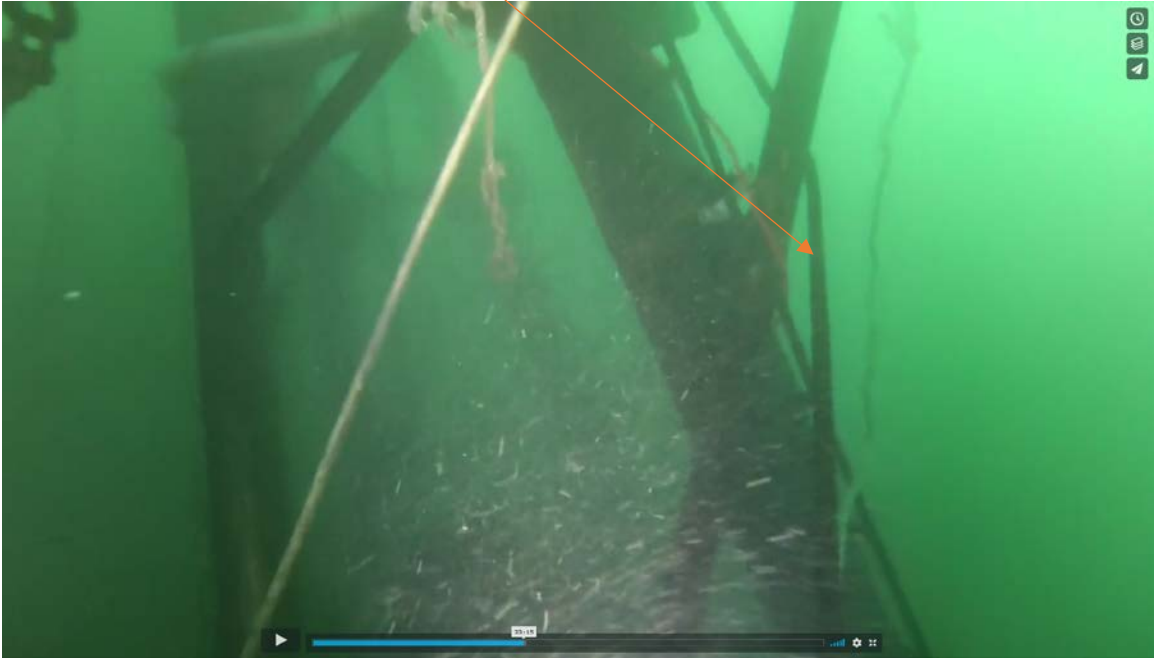
Cable coming from the dredge up to the block
