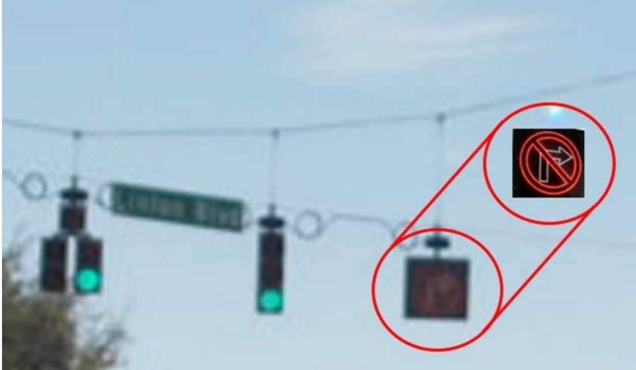
Railroad Signal and Highway Factors Photo 3 – Linton Boulevard grade crossing illustrating figure only prohibition sign indicating “ No Right Turn ” looking to the south. A clear image of the figure only turn prohibition sign indicating “ No Right Turn ” is shown to the upper right when active.
