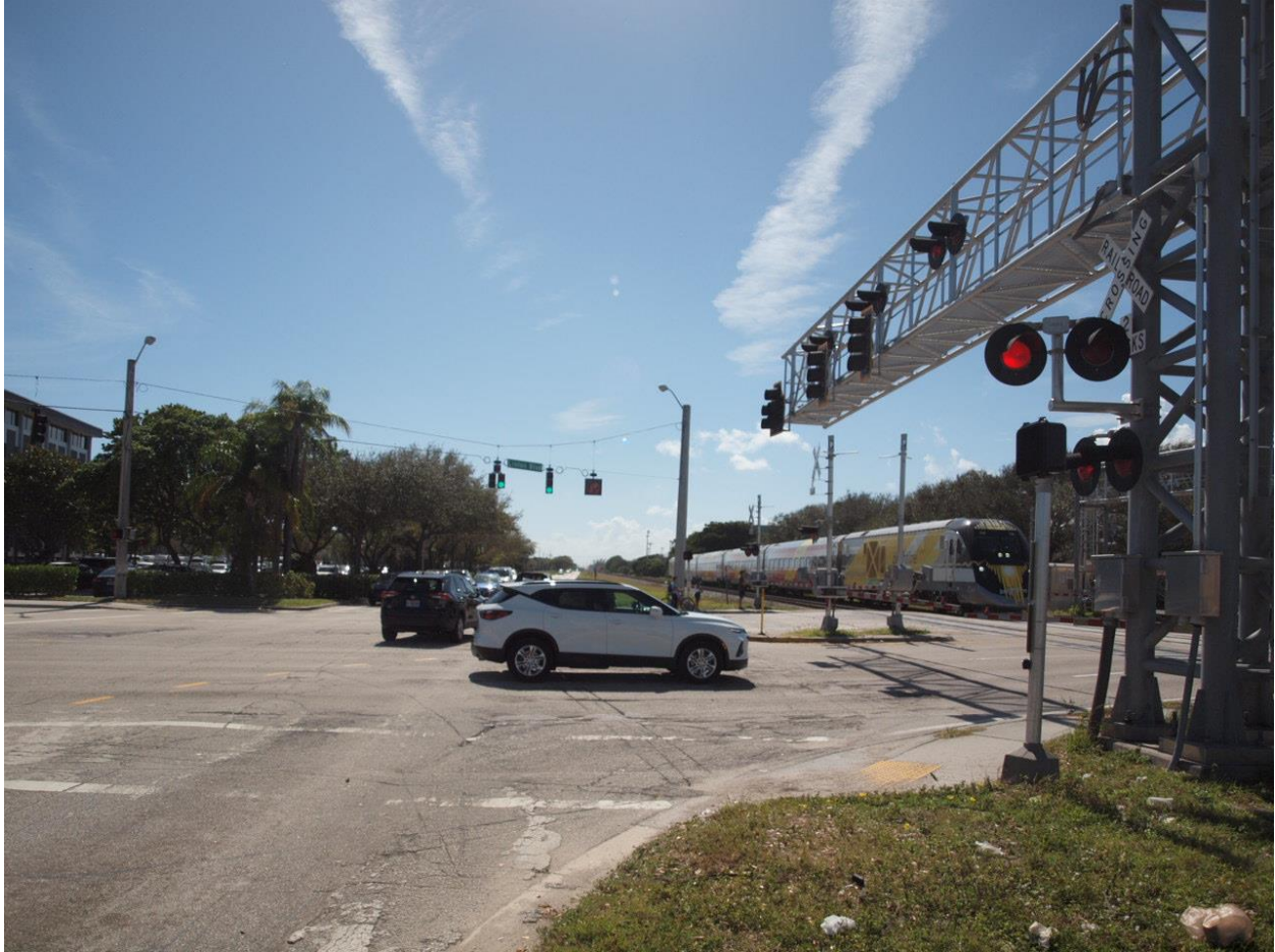
Railroad Signal and Highway Factors Photo 13 – View of southbound Old Dixie Highway on approach to the Linton Boulevard intersection with the Brightline passenger train shown in the background
