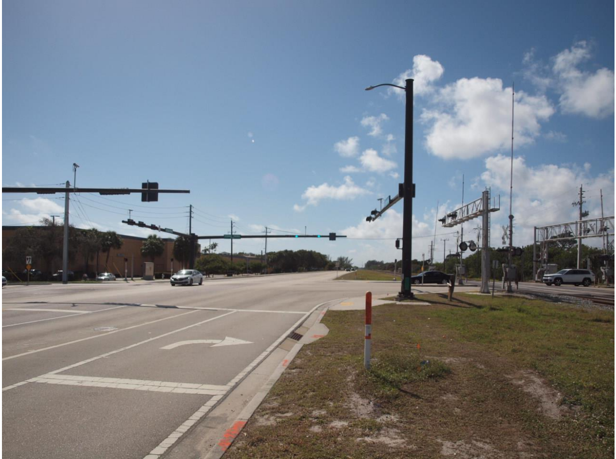
Railroad Signal and Highway Factors Photo 11 – View of southbound Old Dixie Highway on approach to the Hidden Valley Boulevard intersection
