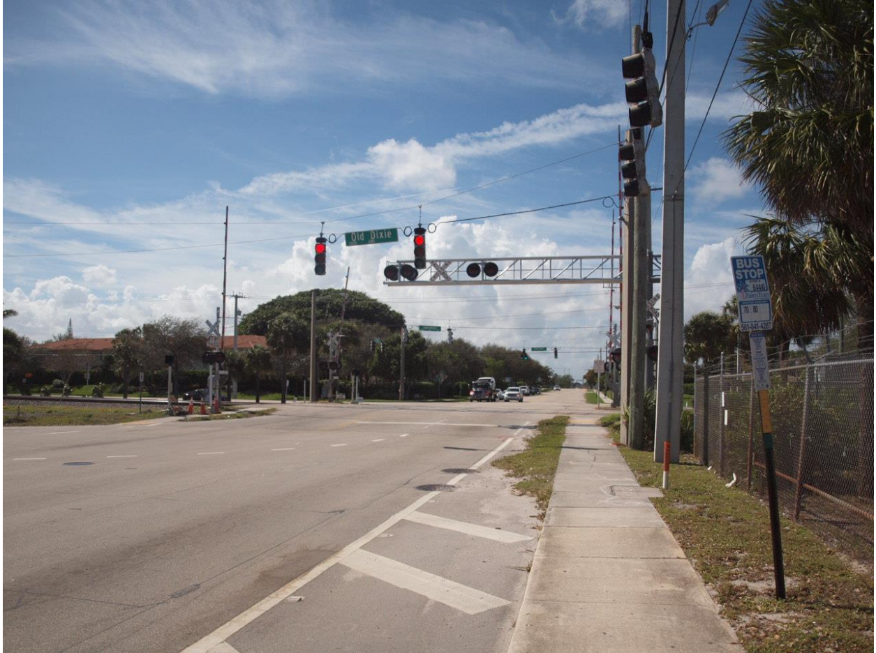
Railroad Signal and Highway Factors Photo 15 – View of westbound S. 10 th Street on approach to the grade crossing
