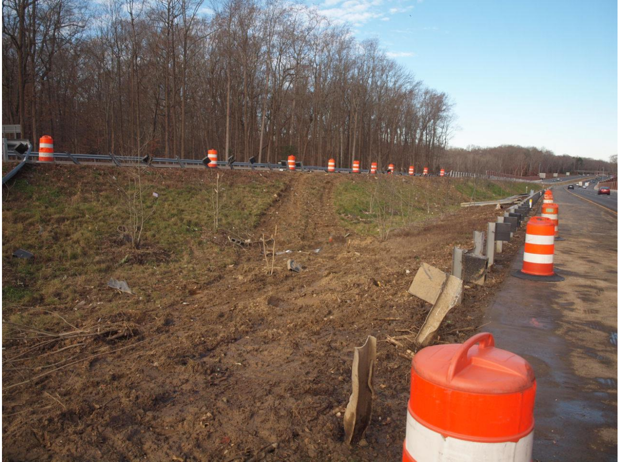
Highway Factors Photo 5 – View of tire marks left in the median by the Freightliner combination vehicle standing in the paved shoulder adjacent to the leftmost travel lane in the westbound direction looking to the northwest
