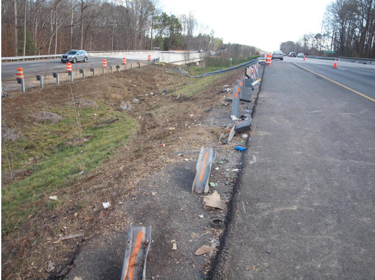
Highway Factors Photo 6 – View of tire marks left in the median by the Freightliner combination vehicle standing in the paved shoulder adjacent to the leftmost travel lane in the eastbound direction looking to the southeast
