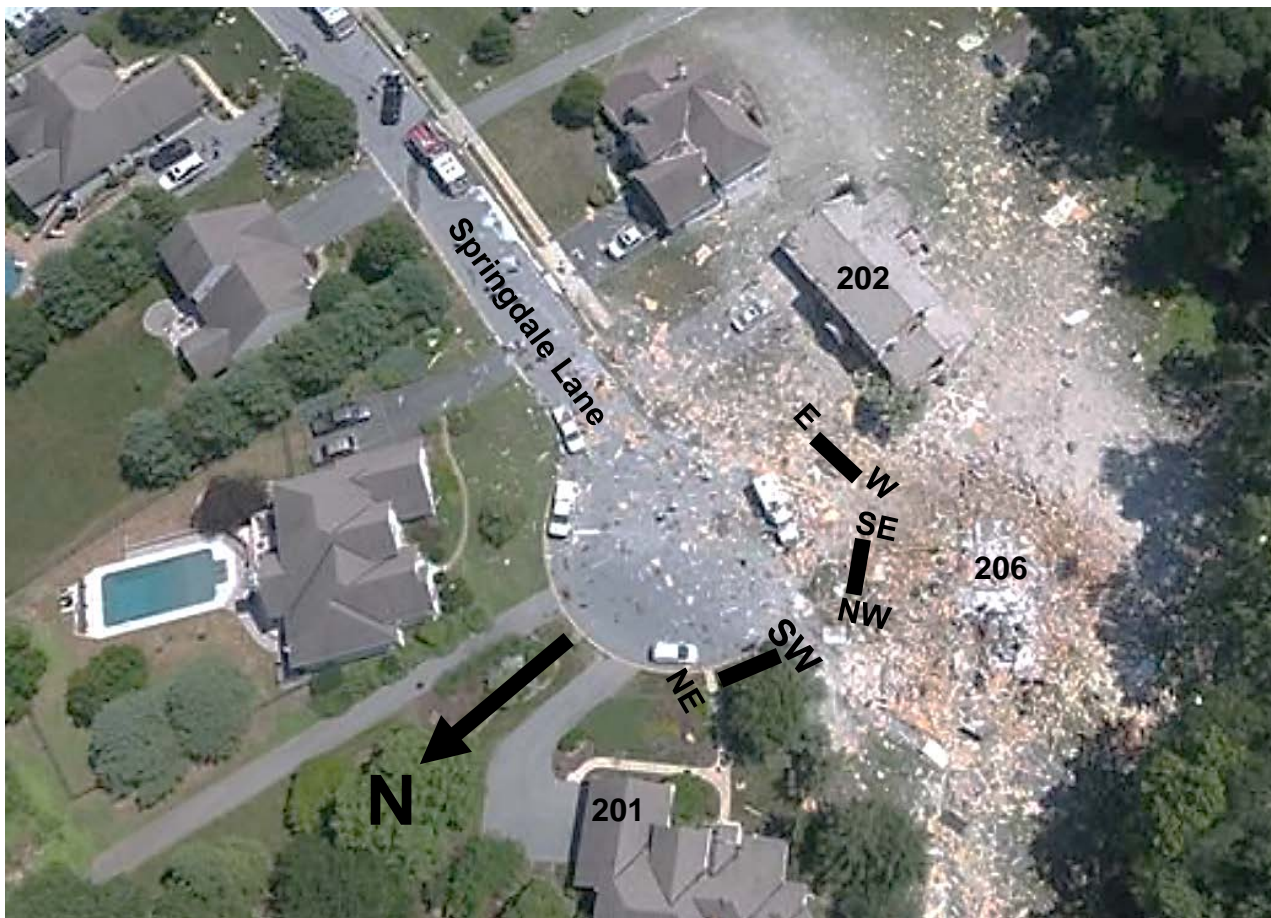
Figure 30. Overhead photograph of the house that was involved in the accident (206 Springdale Lane). Three four-foot long main segments each containing the tapping tee assembly for dwellings 201, 202, and 206, were removed from the accident site and transported to the Safety Board Materials Laboratory. The approximate location of removed gas main segments are indicated by a black line. The cut ends of the gas main segments were labeled with approximate orientation relative to the North (N) direction. For example, the gas main portion in front of dwelling 206 was oriented in the SE-NW direction.
