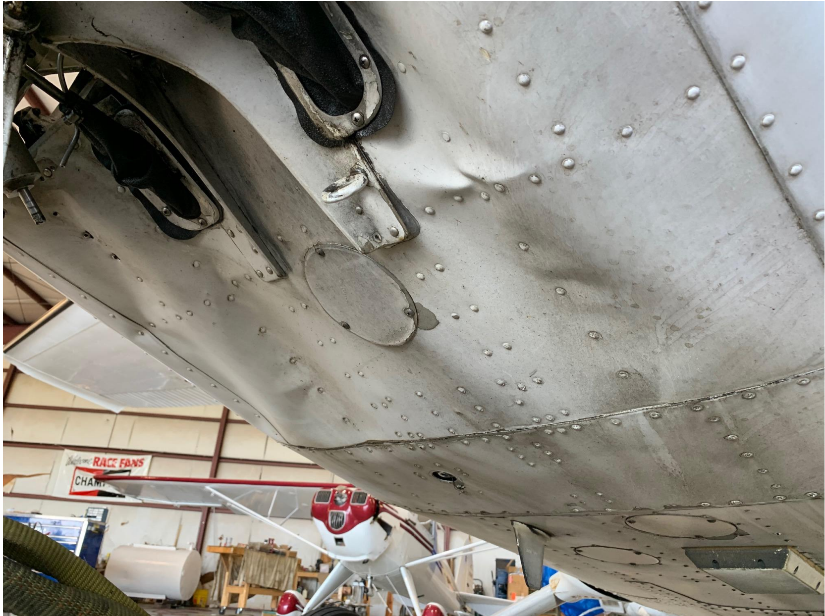
Airplane – View of Forward Fuselage Damage (courtesy FAA)
