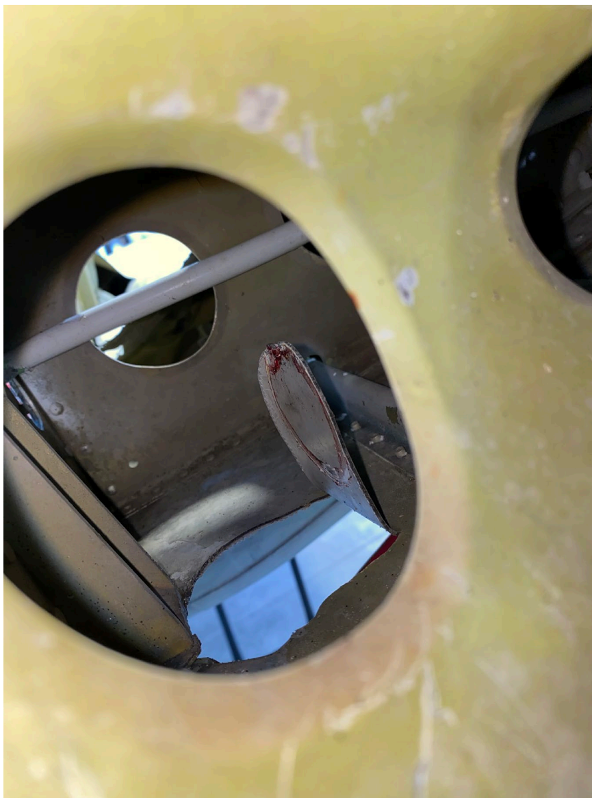
Photograph 4 - Horizontal Stabilizer - Center Lower Panel (Internal)
