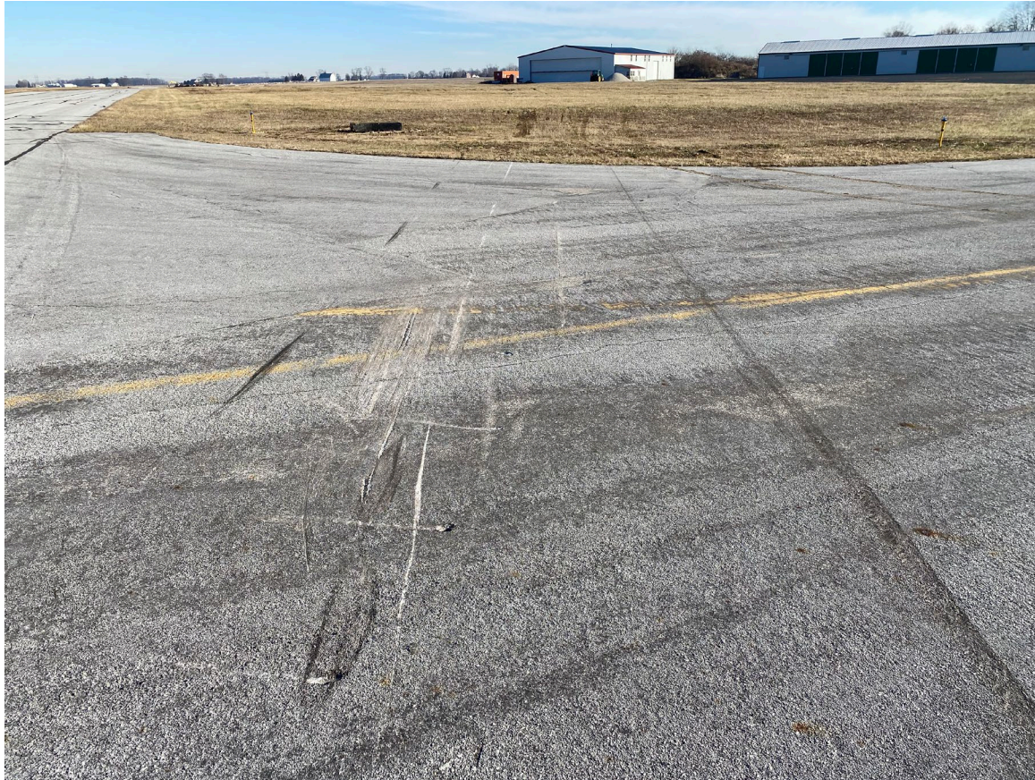
Photograph 4 - Runway/Taxiway skid marks and propeller strikes (Courtesy of FAA)
