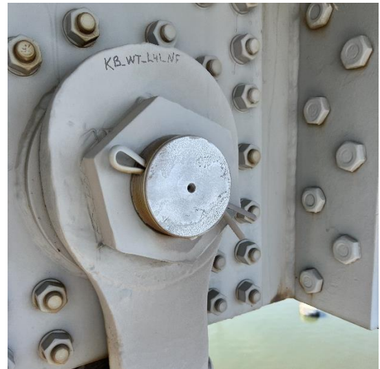
Figure 3: Photo and UT scan showing the headed end pin backwall of West Truss, L41, North Face Pin (Taken from threaded end)
