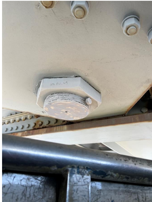
Figure A65: KB-P61-WS (Wind Shear Pin) Bottom Side
