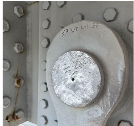
Figure 2: Photo and UT scan showing the nut stepdown, cotter pin hole, and threaded end pin backwall of West Truss, L41, South Face Pin (Taken from headed end)
