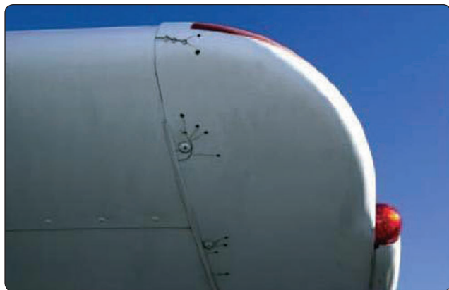
Figure 2-8. Cracks radiating from screw holes that have been stop-drilled to prevent crack progression.
