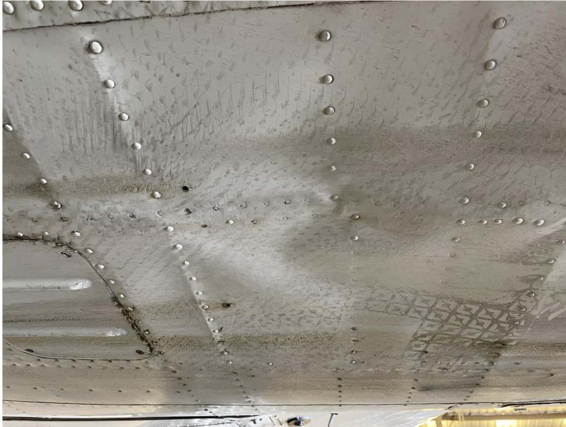
Photograph 3 - Aircraft damage (Courtesy of Airport Operations Manager)
