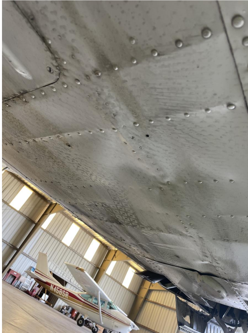
Photograph 4 - Aircraft damage (Courtesy of Airport Operations Manager)
