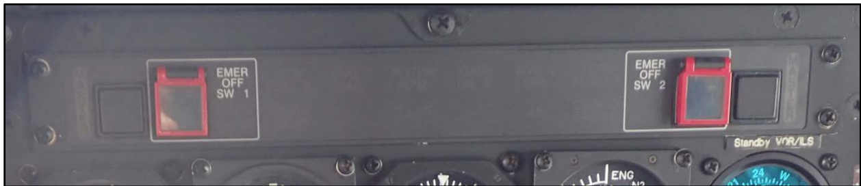
Figure 17 – Exemplar view of the caution and warning unit in N145DU.
