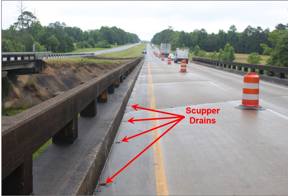
Figure 7: Scupper Drains through Bridge Deck
