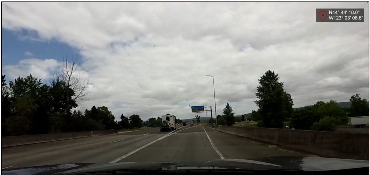
Figure 4: Cantilever supported informational service sign stating "rest area travel info center" with a yellow "exit only" panel located about 170 feet past the ramp gore.
