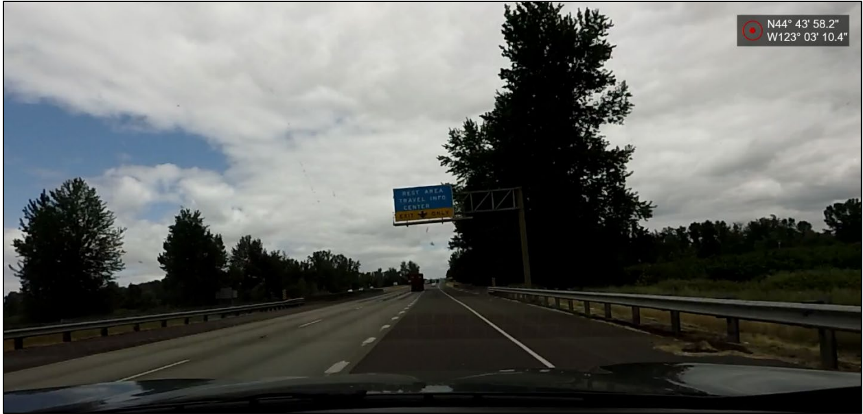
Figure 3: Cantilever supported informational service sign stating "rest area travel info center" with a yellow "exit only" panel located about 1980 feet south of the ramp gore.
