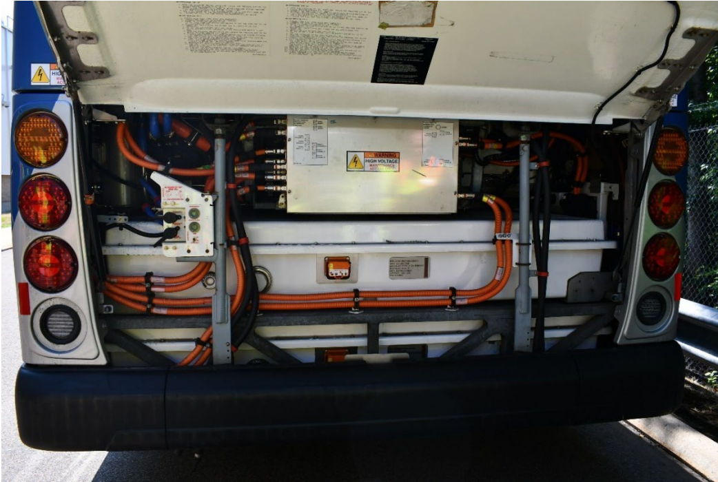
Figure 5: Rear mounted energy storage enclosures on exemplar bus
