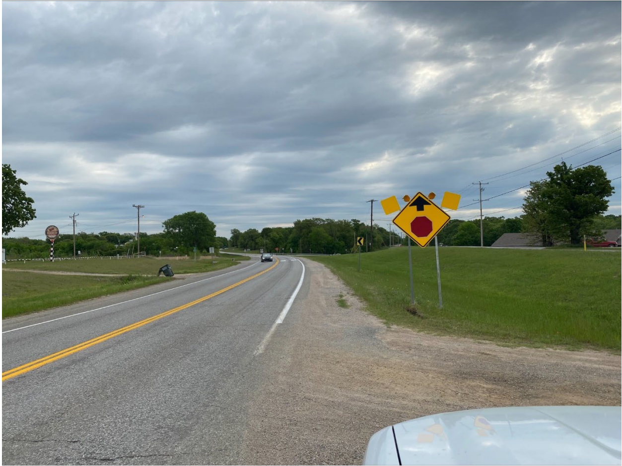
Figure 13. View of the STOP AHEAD advance warning sign equipped with flags on eastbound SH 22. (source: ODOT)
