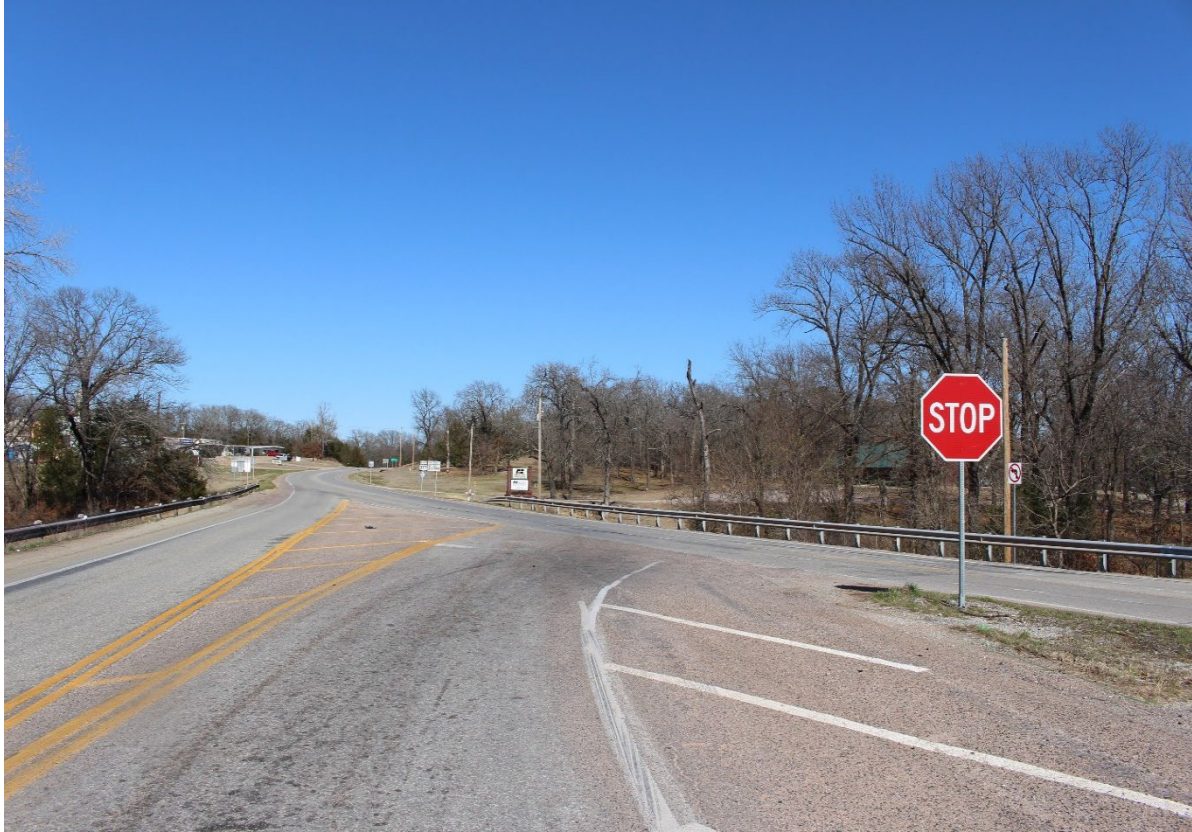
Figure 5. View of STOP sign on eastbound SH 22 at US 377.
