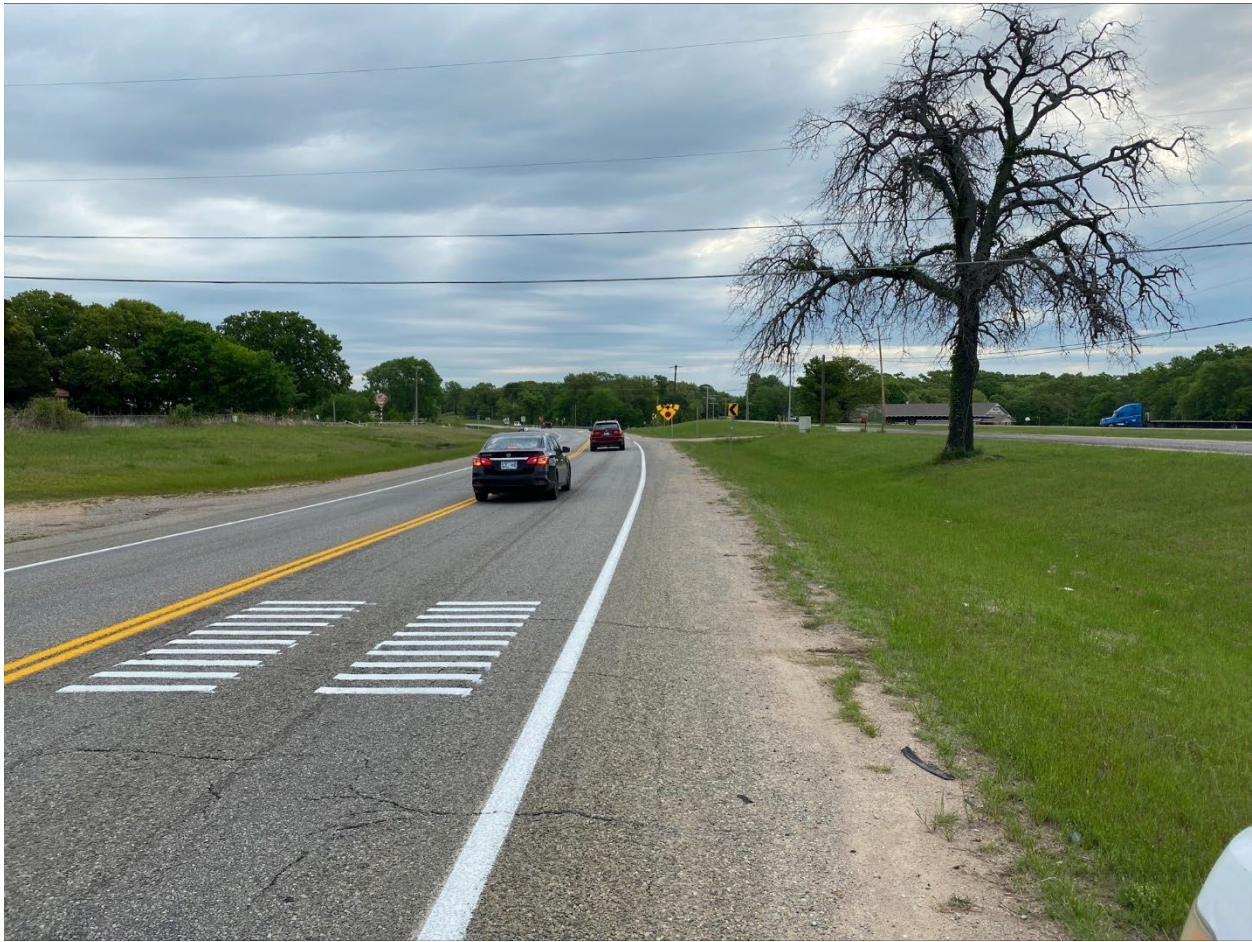
Figure 12. View of transverse rumble strips preceding the STOP AHEAD advance warning sign on eastbound SH 22. (source: ODOT)
