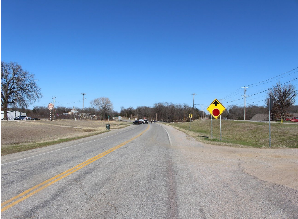
Figure 4. View of STOP AHEAD advance warning sign.
