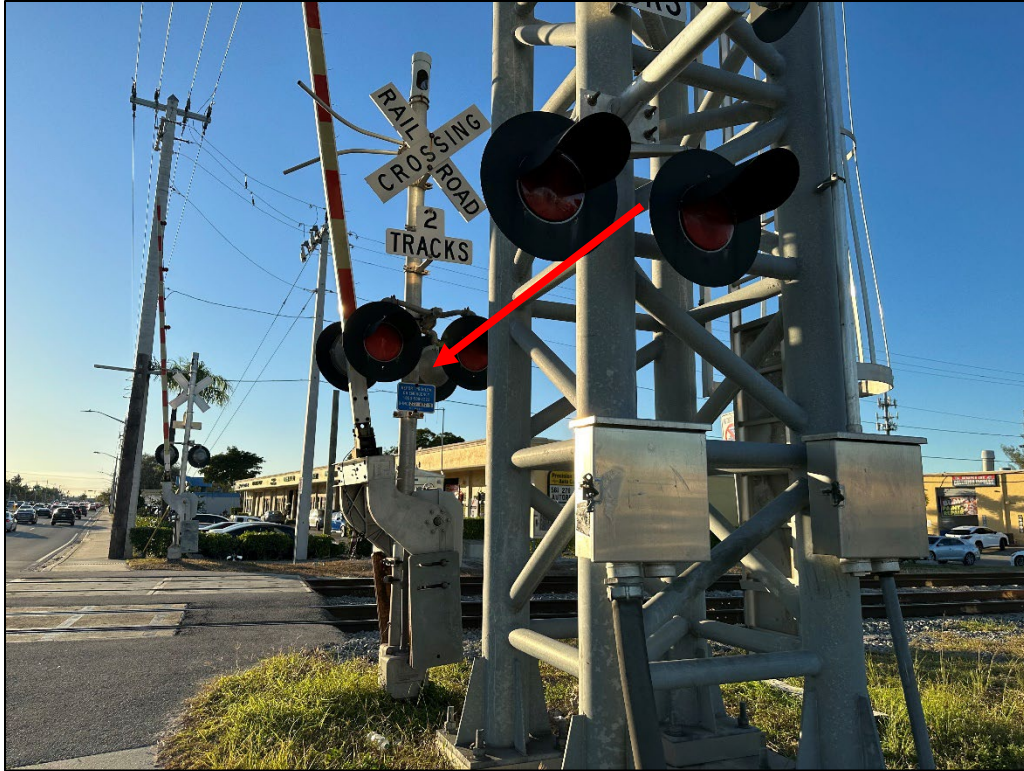
Figure 5: Westbound Linton Boulevard Emergency Signage
