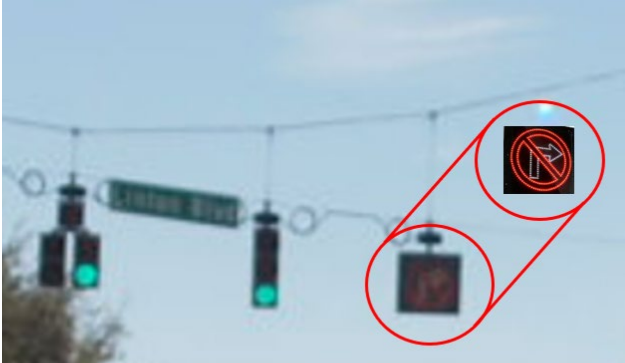
Figure 11 - Linton Boulevard grade crossing illustrating figure-only turn prohibition sign indicating “No Right Turn” looking to the south. A clear image of the figure-only turn prohibition sign indicating “No Right Turn” is shown to the upper right when active.
