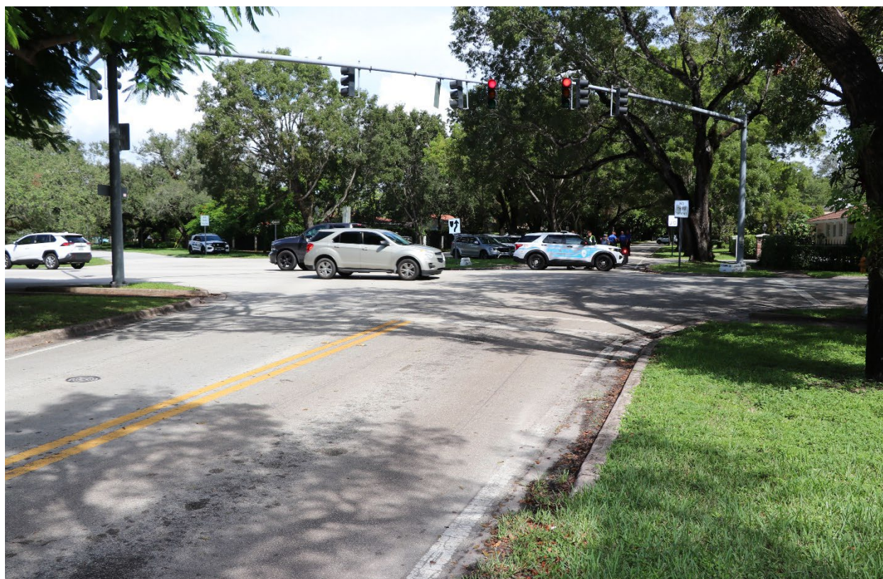
Figure 4: Photograph depicting traffic signals and signal supports looking northbound on Alhambra Circle. (Source: NTSB)
