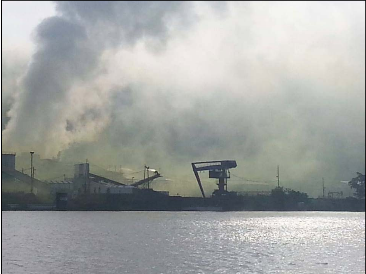
Figure 10 - Close up of the gas leak from the Ohio side of the river
