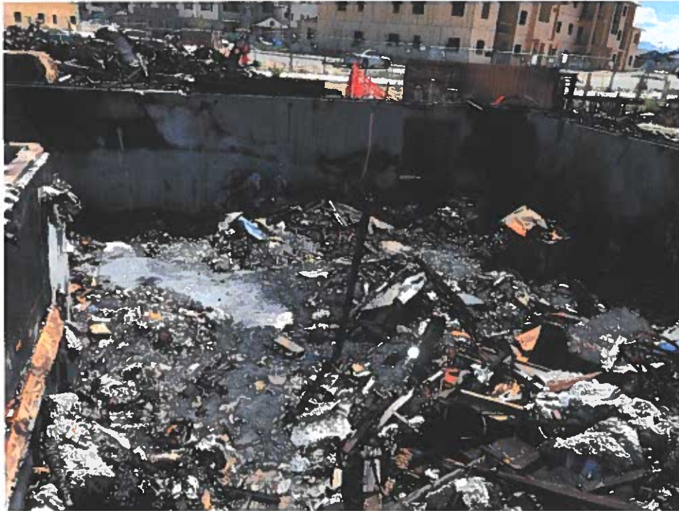
View of basement from ground level.
