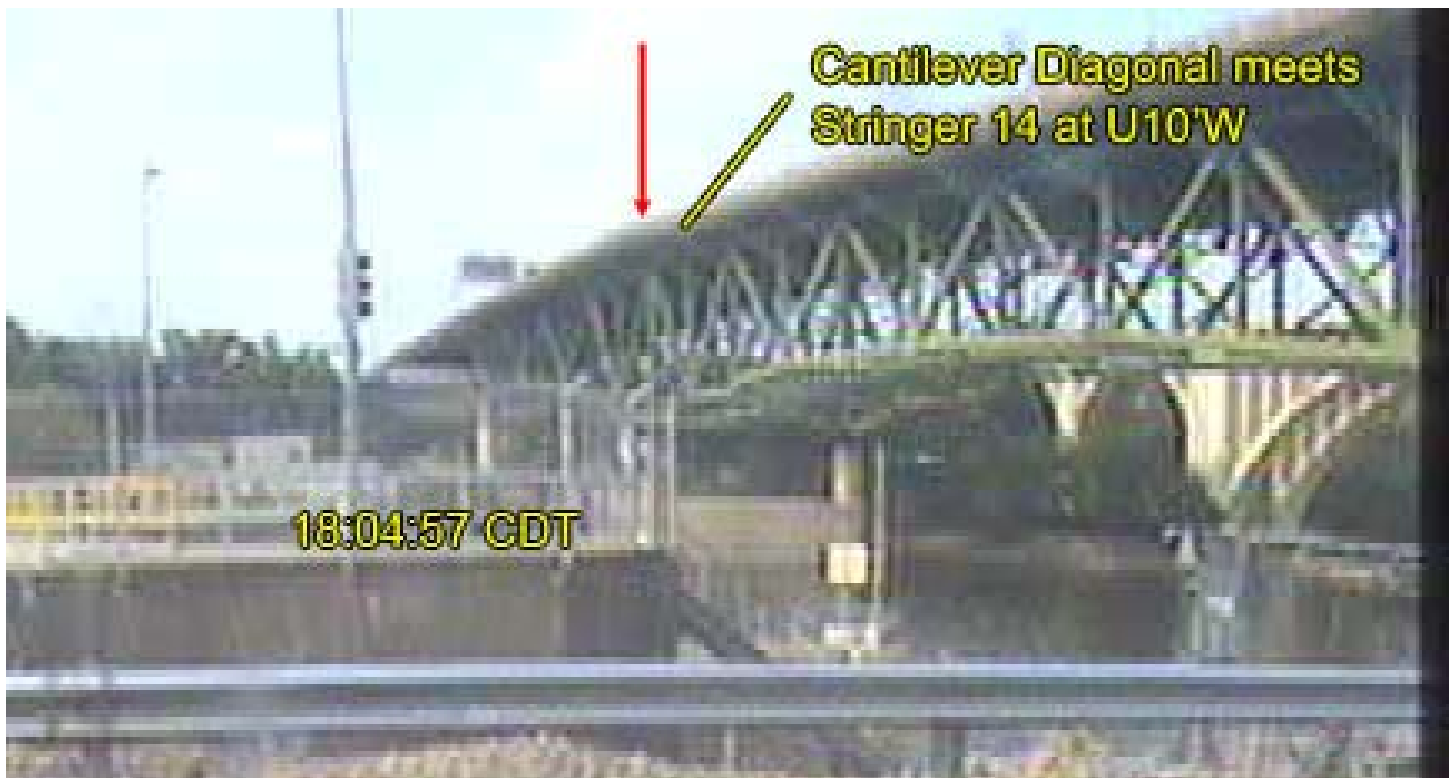
Figure 13. "Bend" in deckline north of U10'W.
