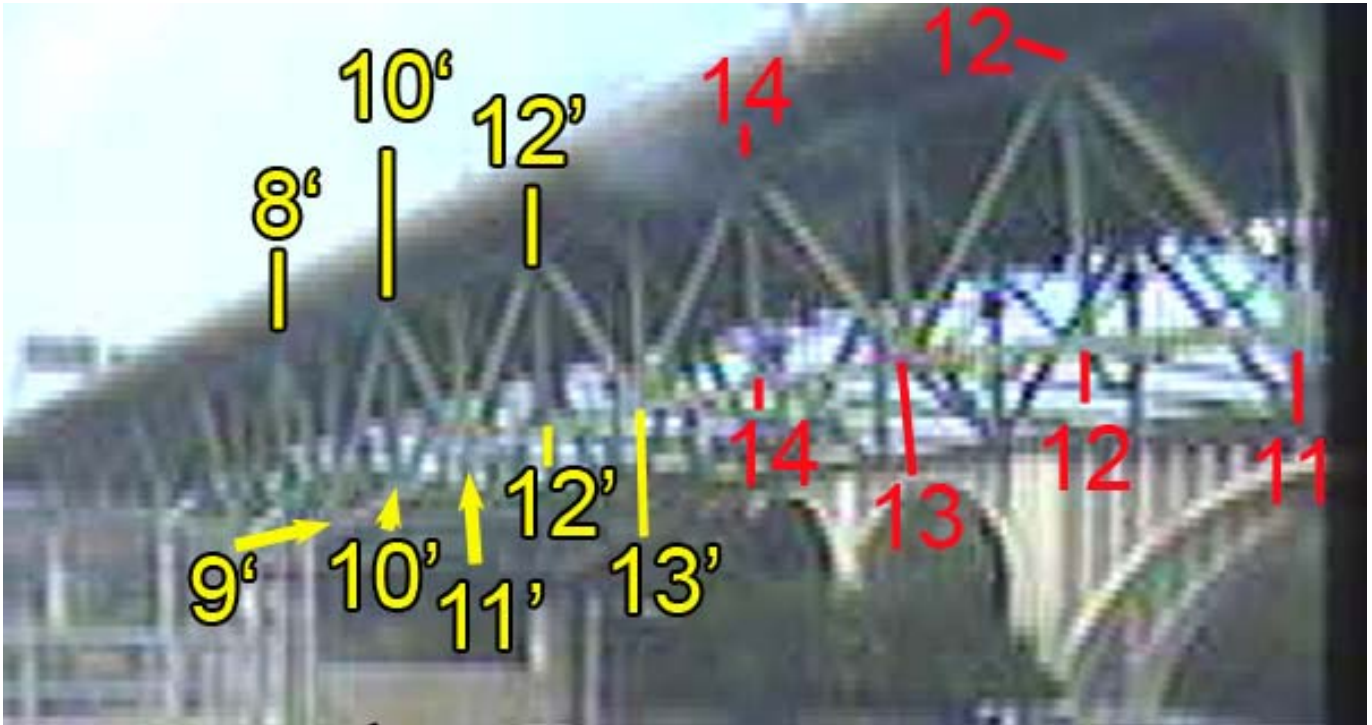
Figure 4. West truss nodes (enlarged view).
