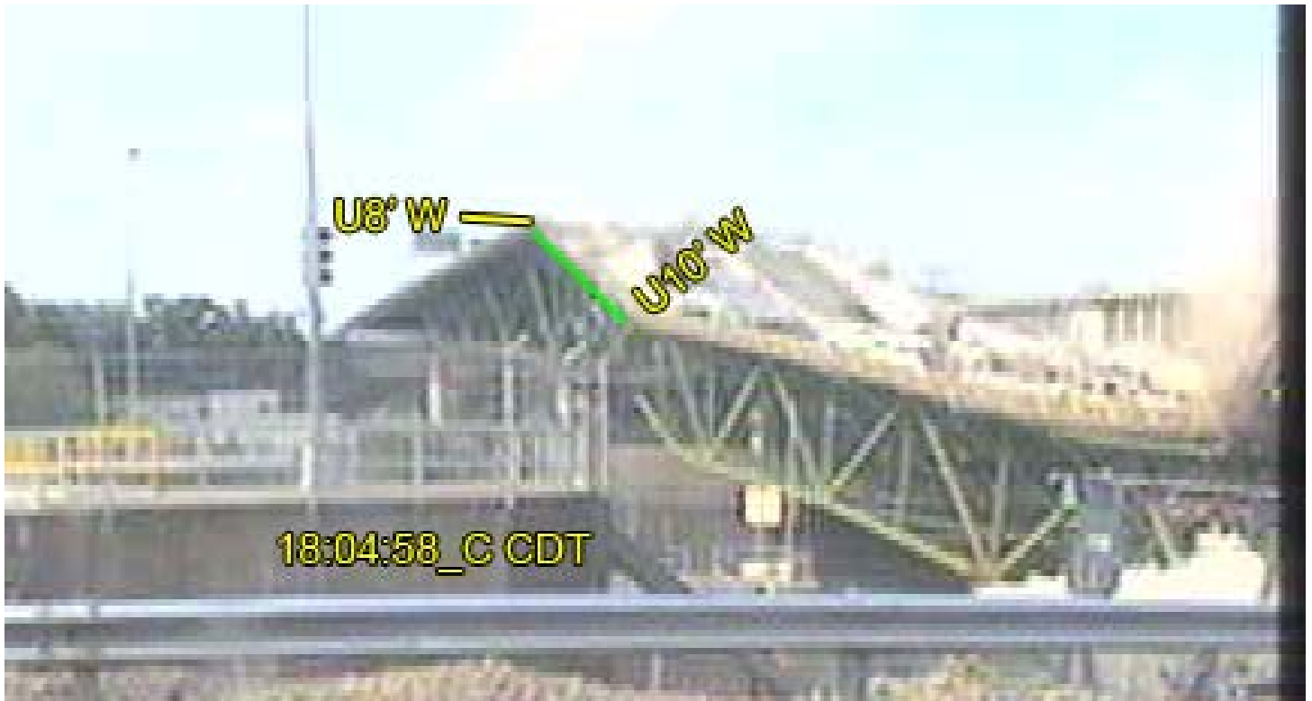
Figure 14. Bridge deck between U8'W and U10'W.
