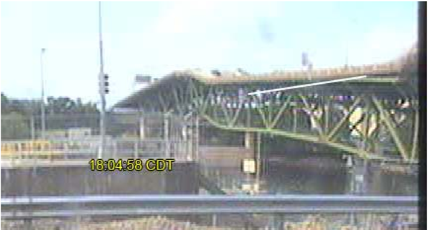
Figure 7. North/south tilt as span 7 fell.
