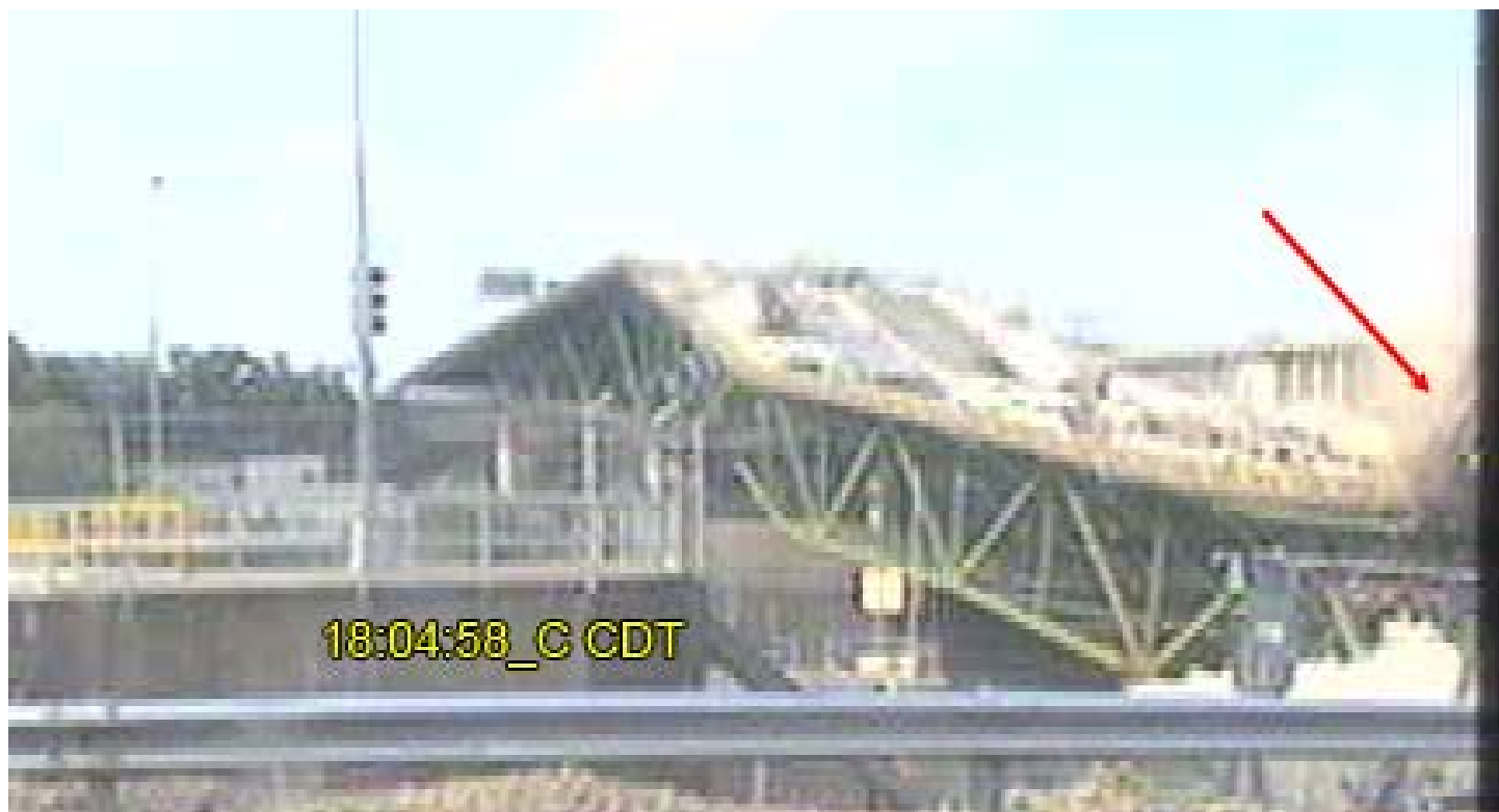
Figure 16. Bridge deck south of node U11W.
