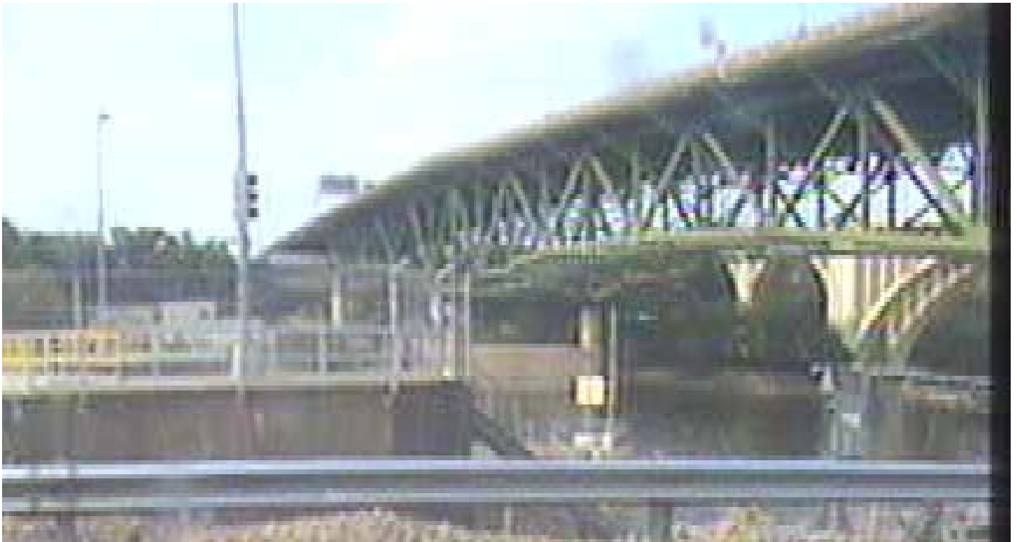
18:04:57 (first image recorded of the collapse).
