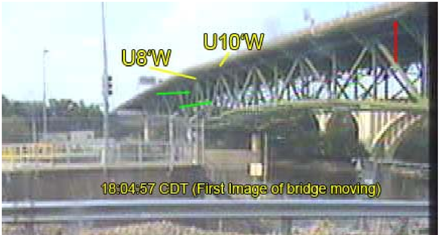
Figure 10. First image of bridge moving at 18:04:57 CDT.
