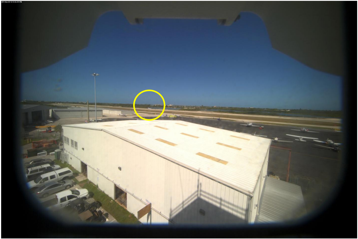
Figure 1 – Camera 1 Northwest View
