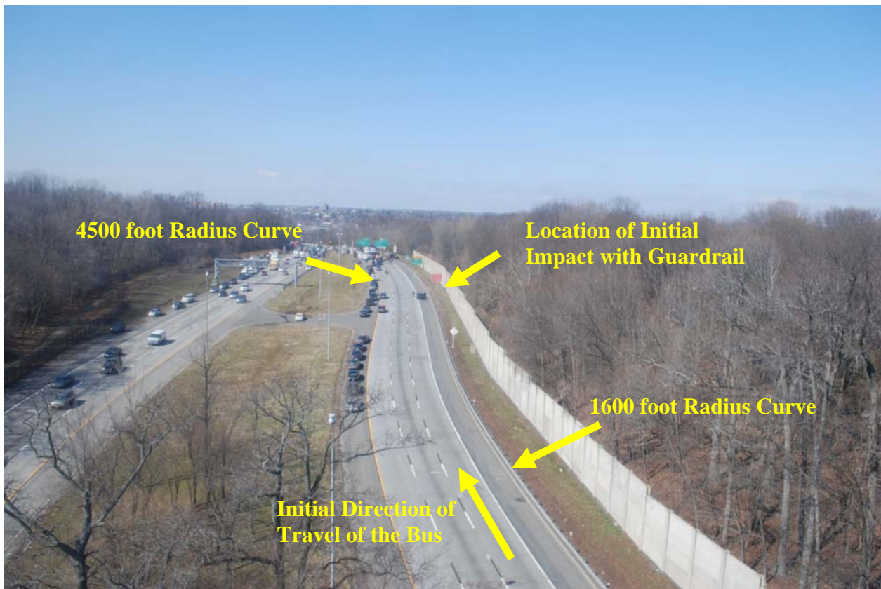
Figure 1 – Aerial view of roadway looking southbound.
