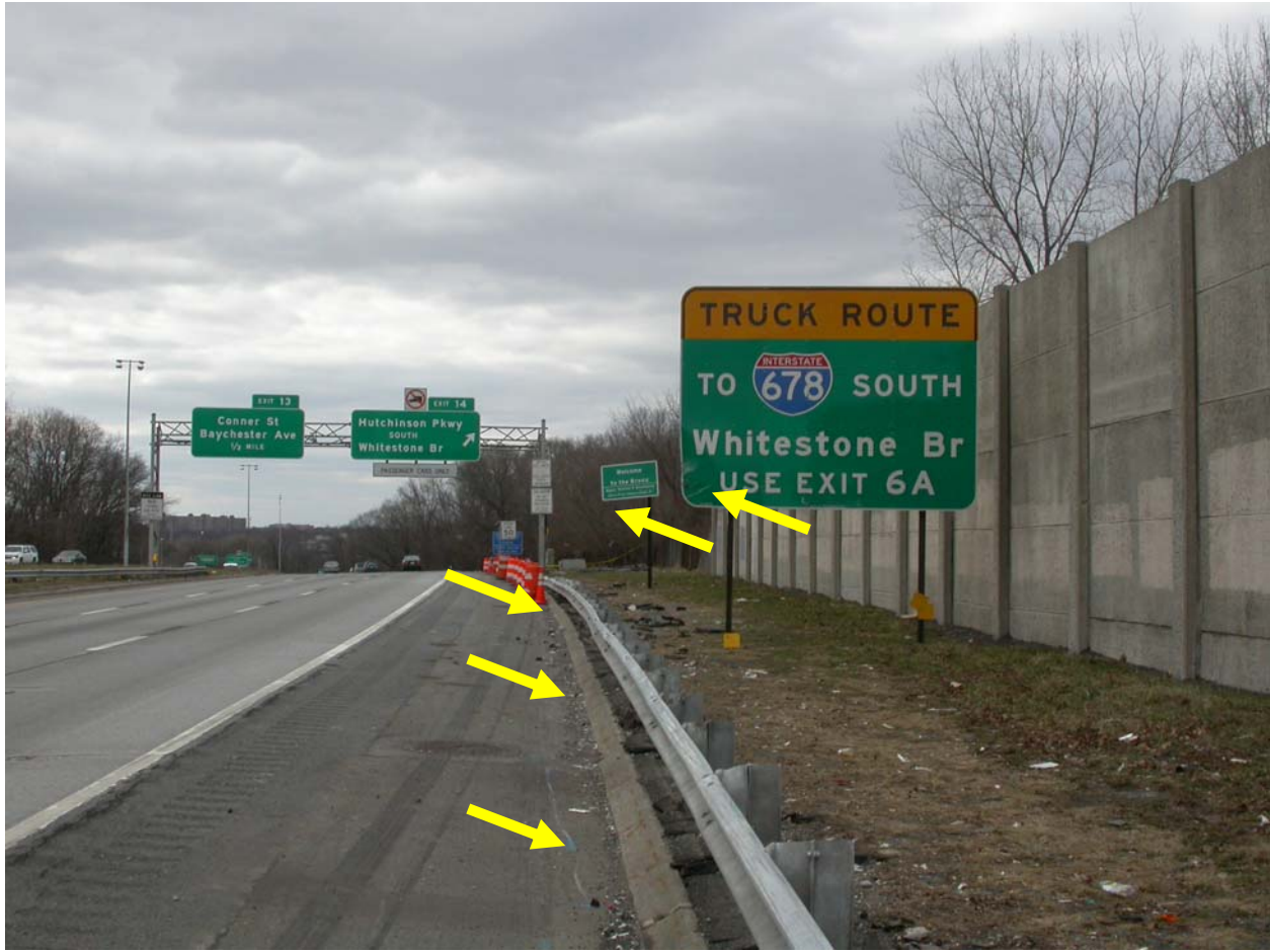
Figure 5 – After striking the guardrail again a second time the bus made contact with the two signs the right of the road shown in this photograph. The arrows on the right highlight damage to the signs caused by impact with bus. Note that the location of the damage indicates that the bus was leaning heavily to the right when it contacted these signs. Arrows on the left point to evidence found on the shoulder indicating the path of the bus after striking the guardrail a second time. Note also the damage visible on the guardrail indicating that the bus was in contact with the guardrail. (Unless indicated by an arrow, tiremarks and scrapemarks shown in the photograph are not associated with this accident.)
