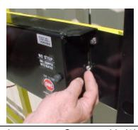
20. Replace cover. Secure with (2) screws. Reseal both ends of the crossing arm cover with RTV. IMPORTANT! – DO NOT seal approximately 1" of the lower right side of the box. This provides an additional drainage location.
