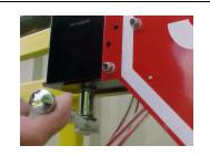
1. Remove ½-20 nut at the bottom of control box w/ 3/4" wrench.
