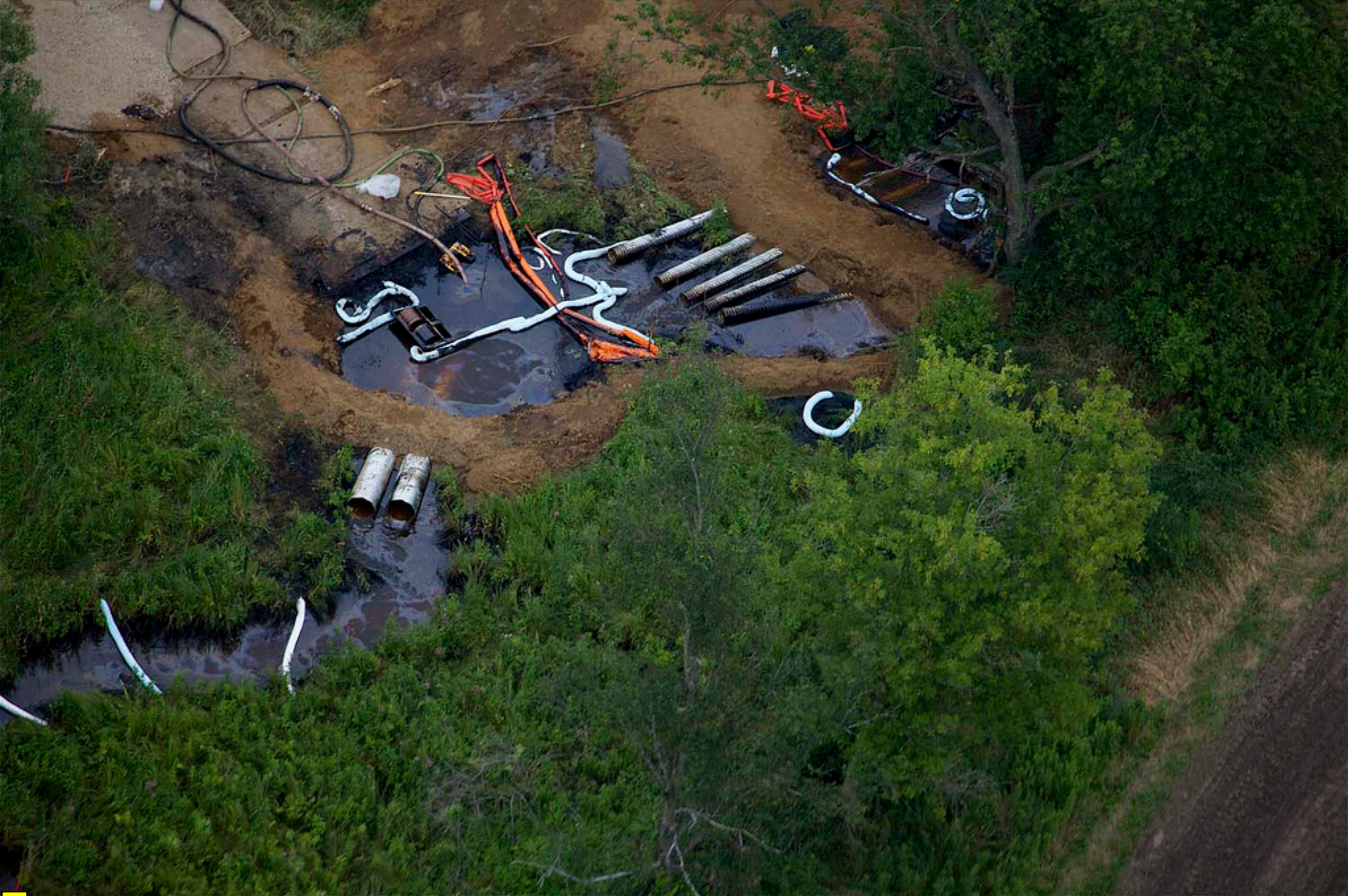
Underflow Dams Constructed on Talmadge Creek, July 30, 2010, State of MI Photo
