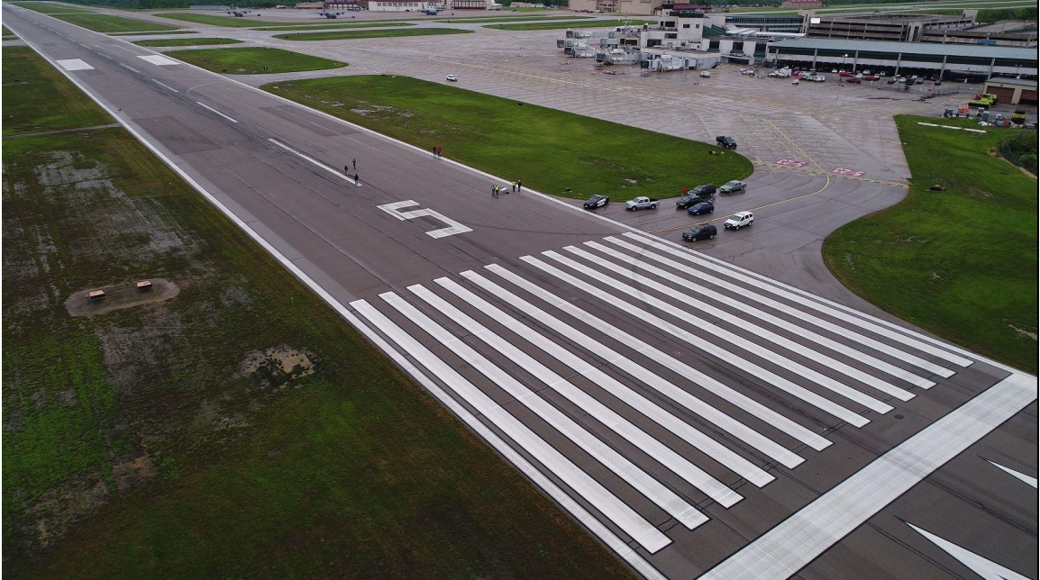
Figure 5 - View of approach end from approximate aircraft position at 150 feet agl
