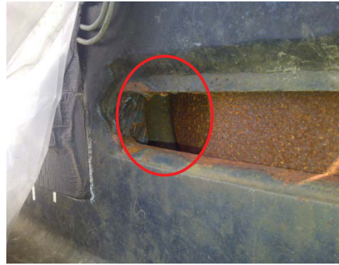
Figure 145: Sill after modification.
