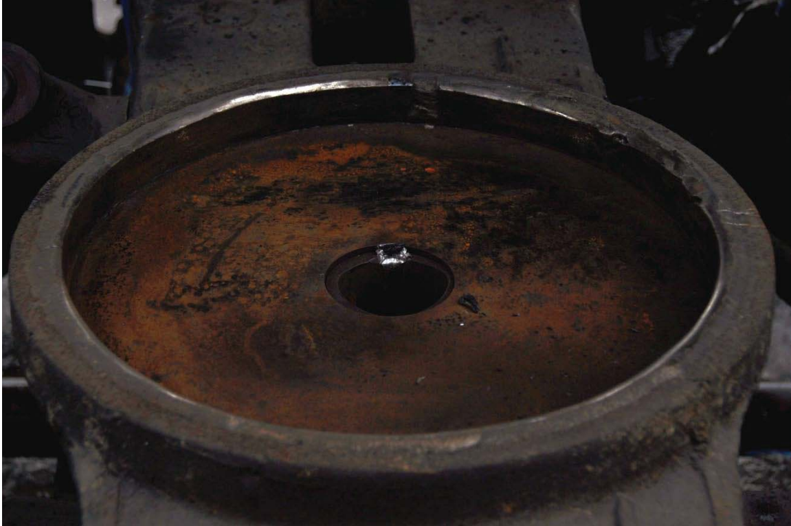
Figure 89: Damage to Car #III centre bowl on near truck.
