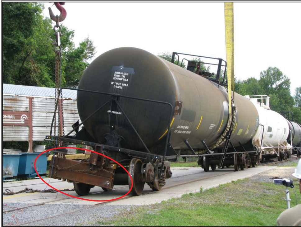
Figure 36: Pulling vertically at the end of the car using a custom-made beam.
