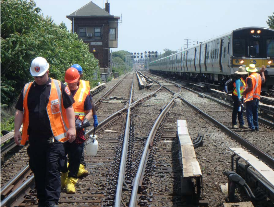
Figure 2. Photo showing accident location taken facing east toward direction of accident train approach.
