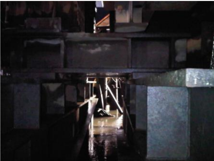
Photo B11. Double bent (toe bent and bent 4) looking west
