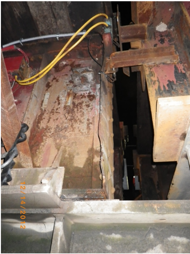
Photo B12. Northeast bearing bent – swing span, east girder
