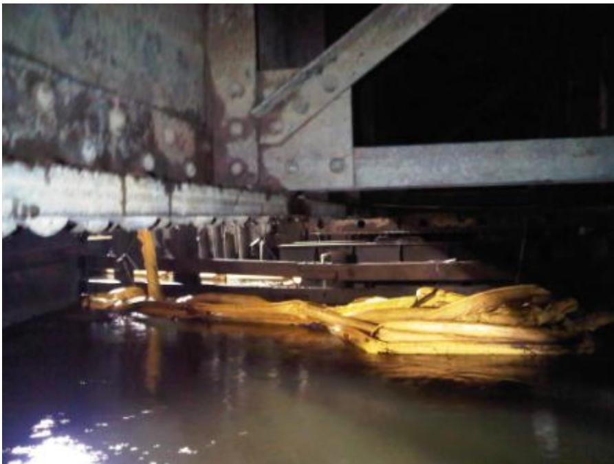
Photo B14. Swing span west girder bottom flange
