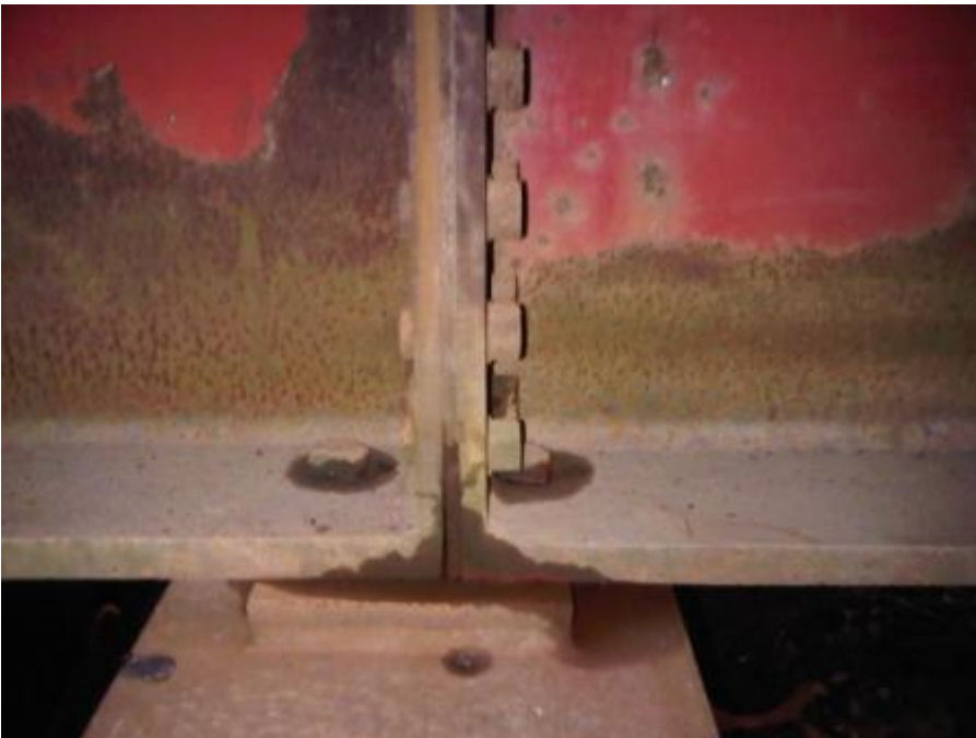
Photo B4. West expansion bearing on Bent 1
