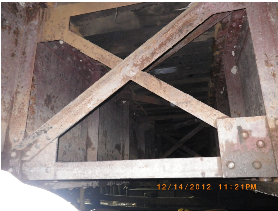
Photo B13. Internal bracing – swing span looking north
