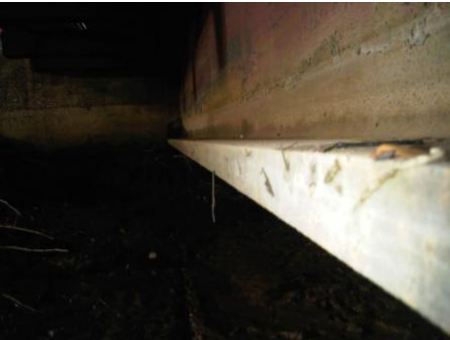
Photo B7. West girder bottom flange, span 4
