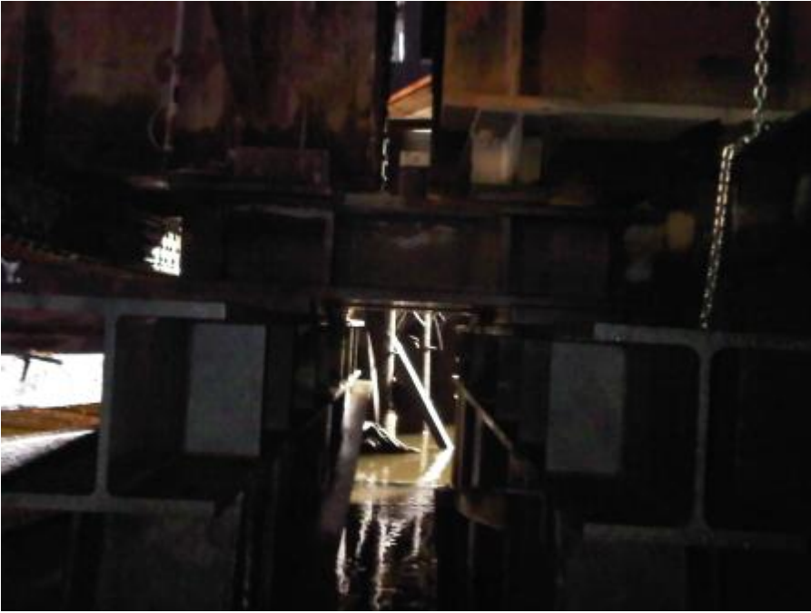
Photo B10. Double bent (toe bent and bent 4) looking west
