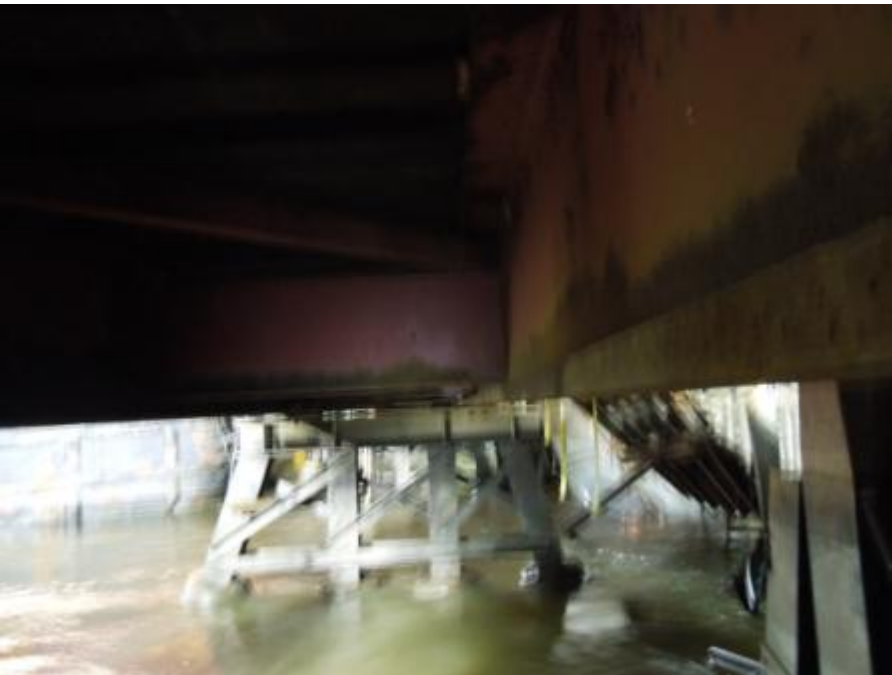
Photo 2. East girder, span 2
