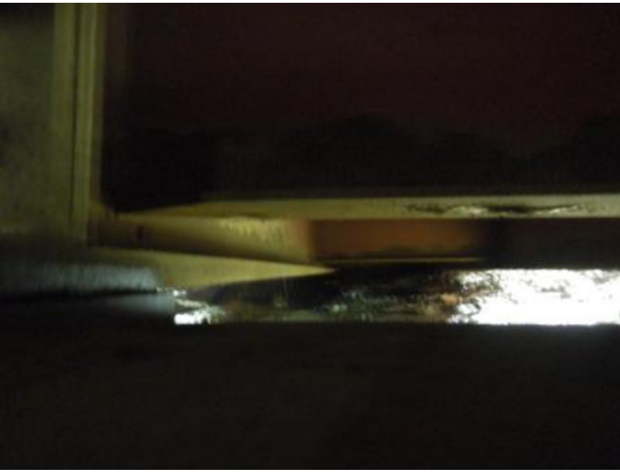
Photo 1. East girder bottom flange, span 1
