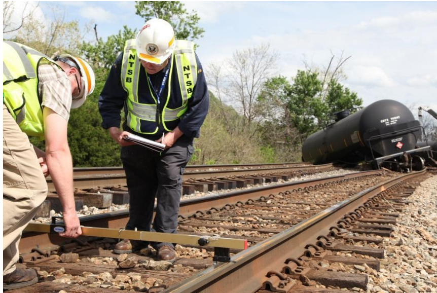
Figure 5. A view looking east at the last car derailed in the background while investigators are taking measurements of the track geometry.
