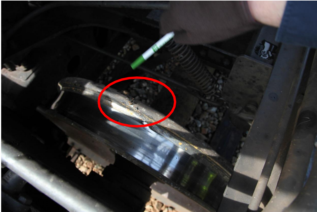
Figure 2. A close-up view of the wheel flange strike mark observed on the 34 th car's rear truck, rear axle, the L1 wheel.
