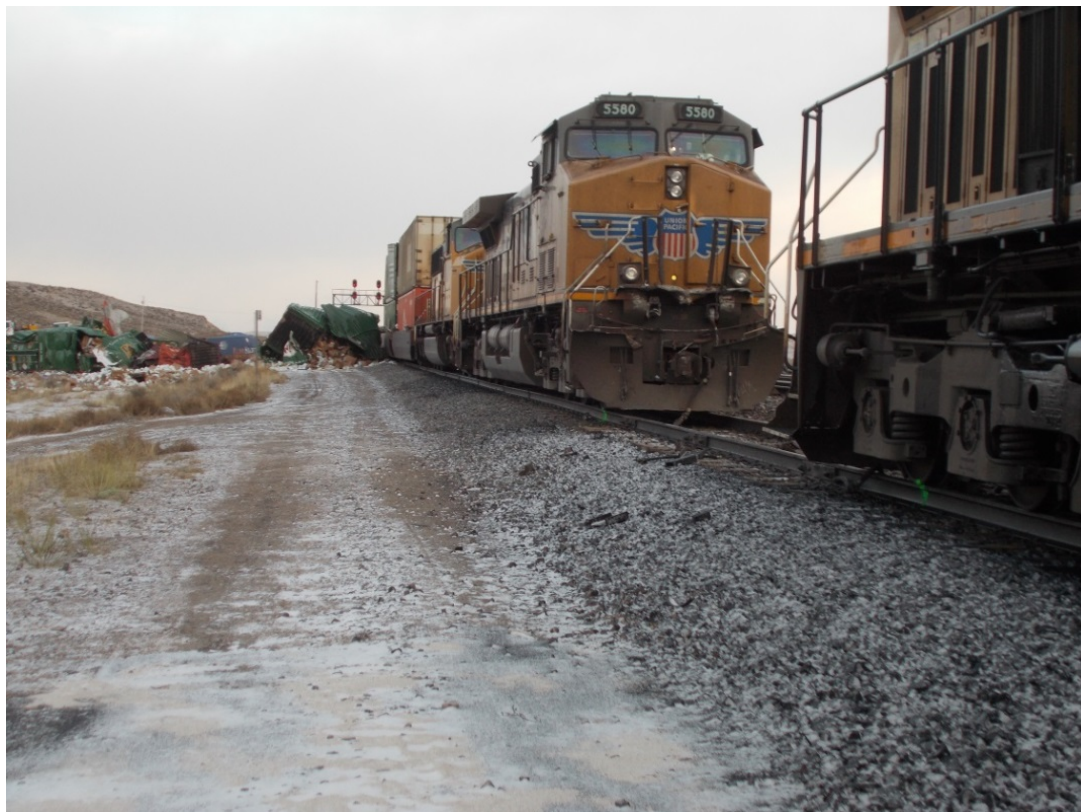
Figure 2. This is a view looking east at the intermodal train derailed cars.
