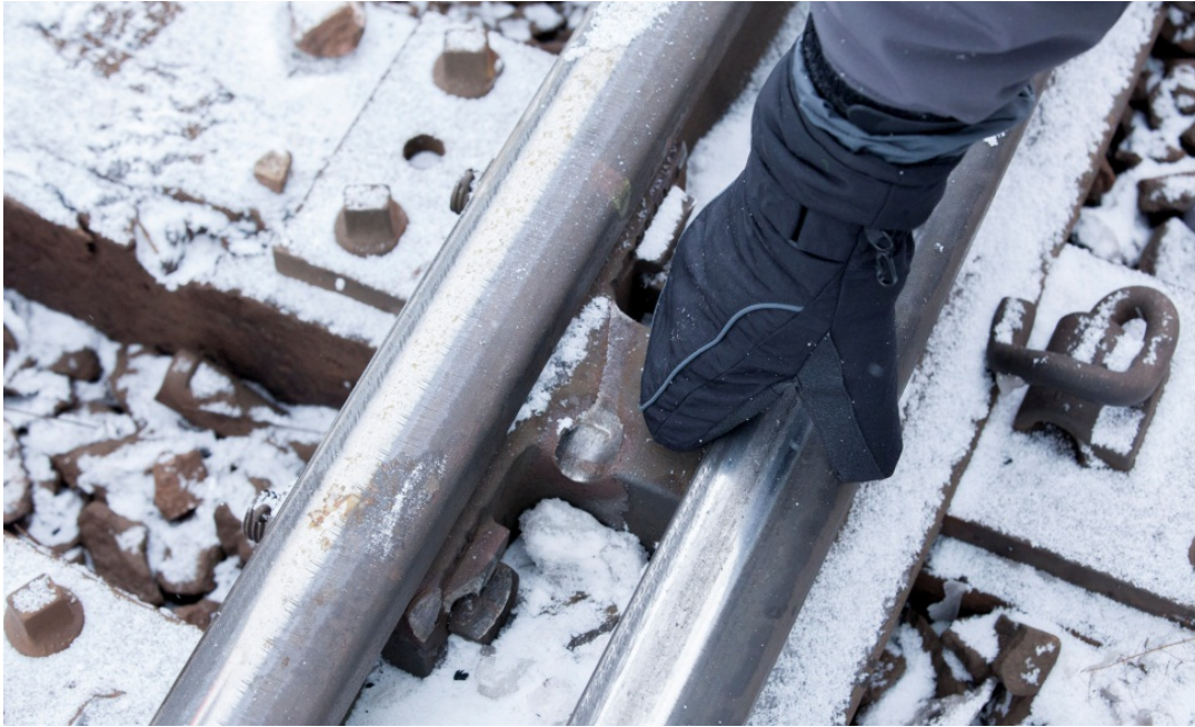
Figure 5. Strike mark located at left hand switch point heel block
