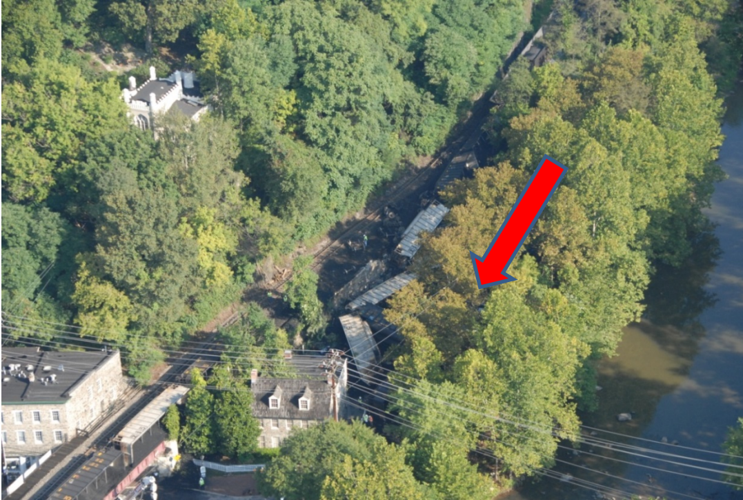
Figure 1. This is an aerial view looking west at derailed coal hoppers along side a railroad track. In the lower left hand corner, one can see the bridge over Main Street in Ellicott City.
