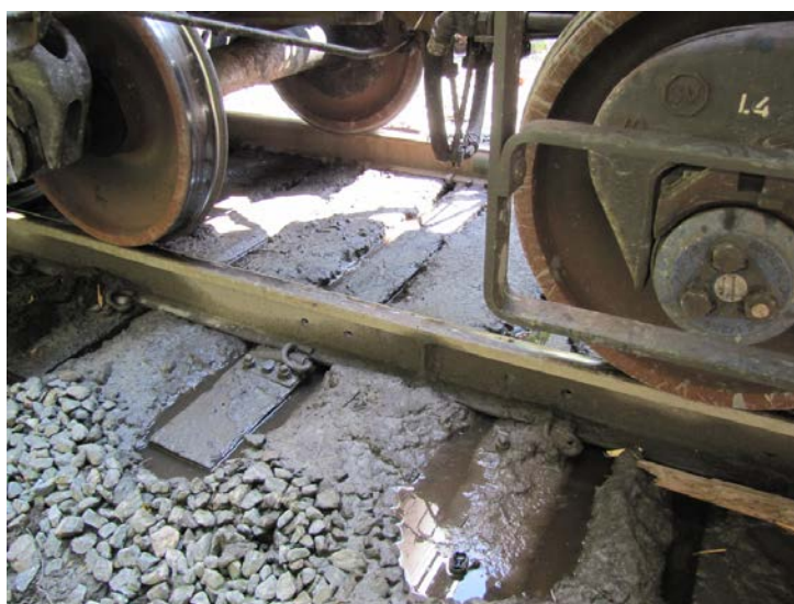
Figure No. 7. View of water and mud condition under derailed car.
