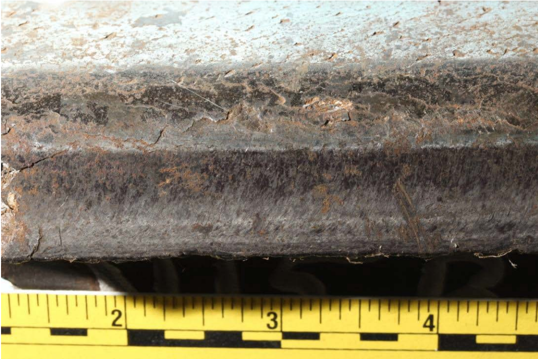
Figure 15. Views of the rail surface on two of the pieces showing rail surface conditions observed on the rail pieces. Unlabeled arrows in the upper image point to some of the cracks associated with surface rolling contact deformation as observed on the running surface near the gage corner.
