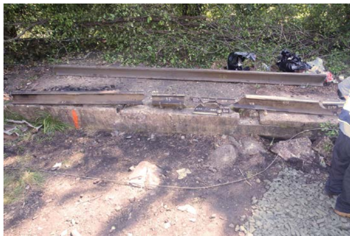
Figure No. 5. View of rail re-build.
