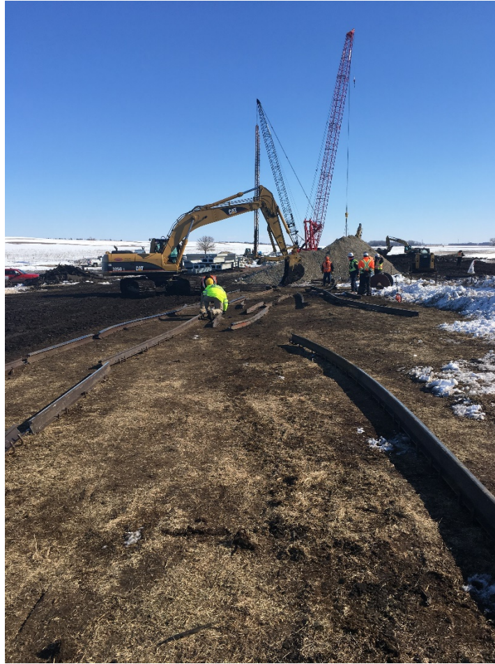
Figure 5-Photograph of rail rebuild.
