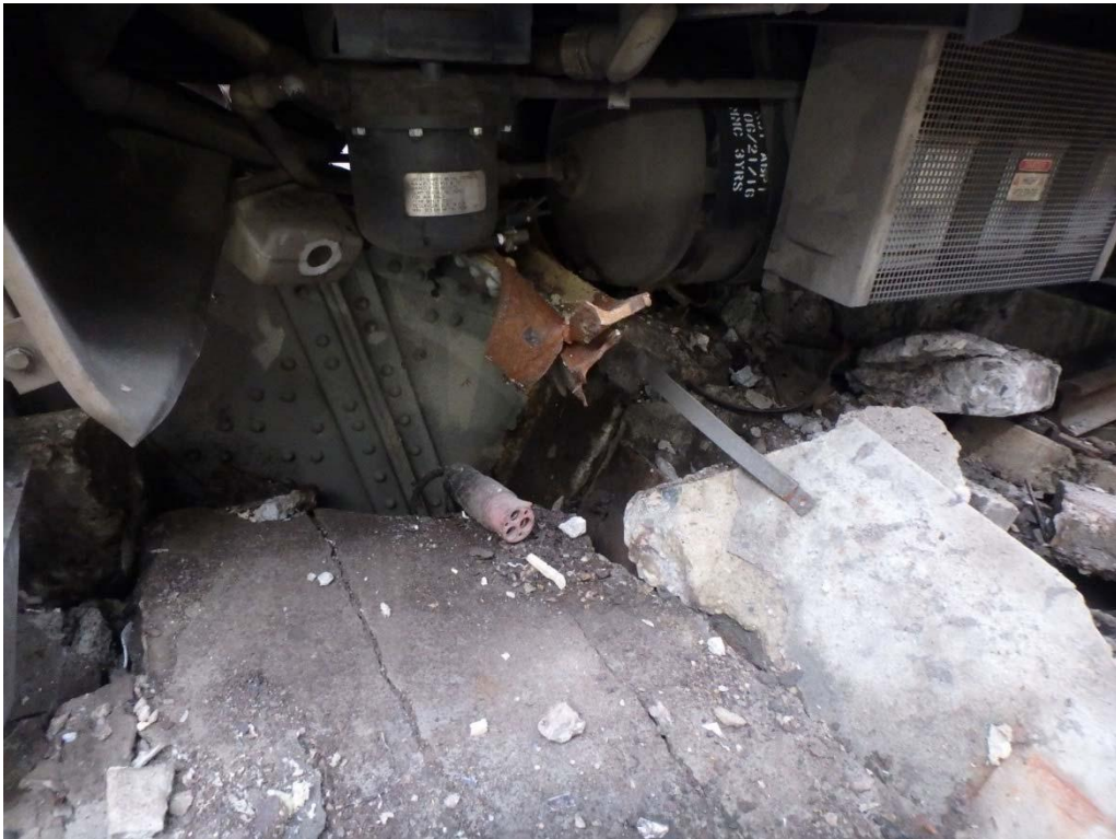
8 9 Figure 5. Photo of track Five bumping post under the controlling cab car. The displaced bumping 10 post and cracked/broken station floor are shown. (Photo NTSB)
