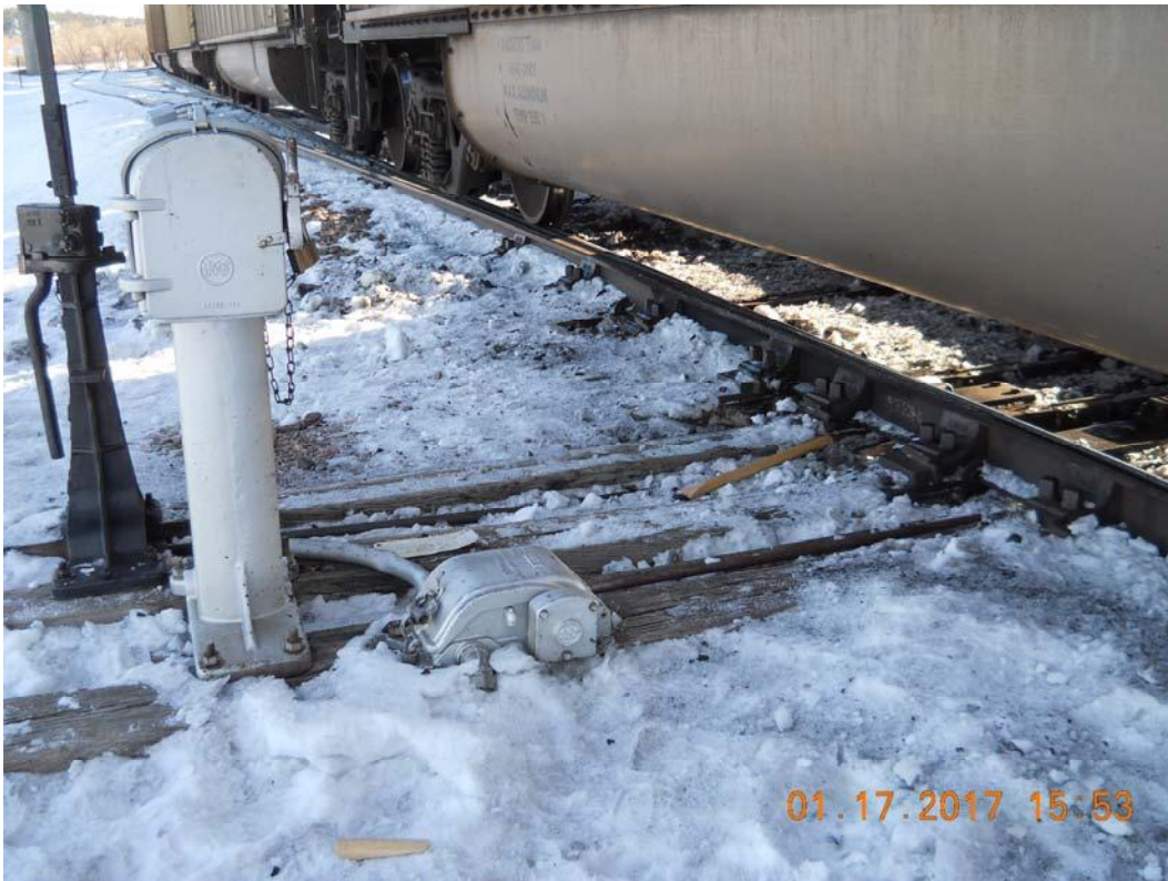
9 10 Figure 1. Switch at west leg of Deadwood Wye.
